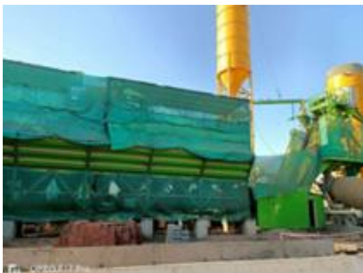
Green net is provided on aggregate bins and silos at batching plant in C5 package
