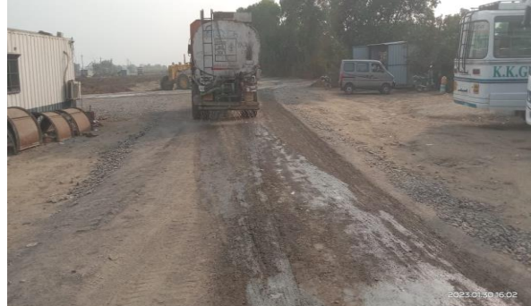
Water Sprinkling is carried out at Surat Station chainage 264.
