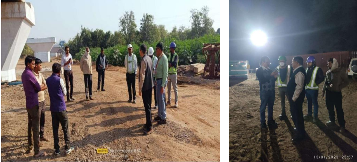
Figure 52: Inspection by Project staff, NHSRCL, Industry representative, GPCB official
