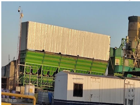
Covershed provided to control dust emission in hoppers at C6 package
