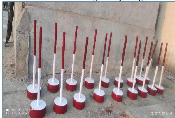
Waste concrete & MS pipes are used for making delineators, Package C4.
