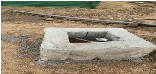
Earthing Pit Developed from Waste Concrete Cube in C8 Package
