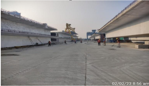
Housekeeping at chainage 188 CY
