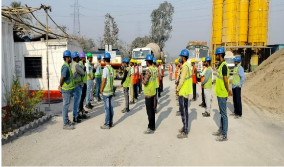
Awareness created about impact due to air pollution at Chainage 165 & 167
