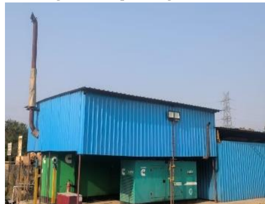
Standard stack height provided to DG in C4 package
