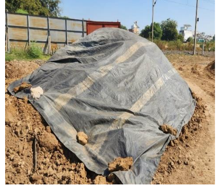
Muck covered with tarpaulin
