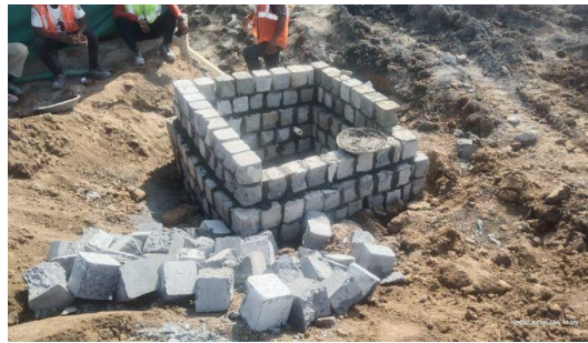
Tested cube used for making water storage taank, garbage Storage zone , drain & chamber in C4 Package
