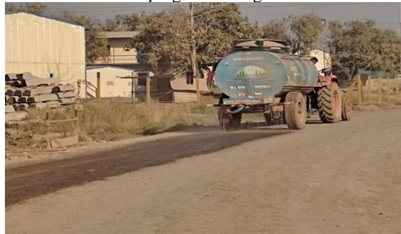
Water Sprinkling is carried out at chainage 165.
