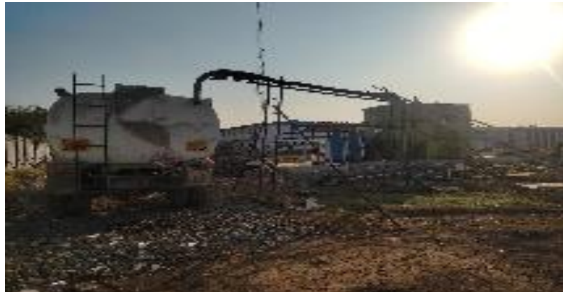
Treated wastewater filling in tanker for using in water sprinkling.
