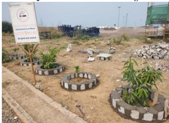
Tested concrete cube is used for making tree guard, Package C4.
