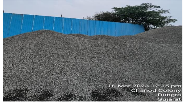
Wind shield provided around Batching plant at Ch. 167
