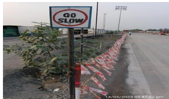
Vehicle speed limit board displayed in PCY 264 to reduce the fugitive emission
