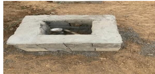
Earthing Pit Developed from Waste Concrete Cube in C8 Package
