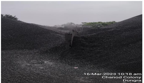
Water Sprinkling at Aggregate storage area in CY 167
