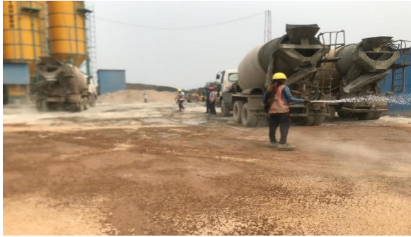
Water Sprinkling at Internal road at Ch. 167
