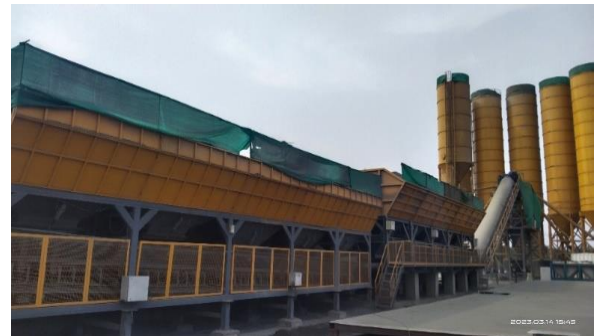
Green net provided to arrest the dust from hopper and conveyor belt at Ch. 217
