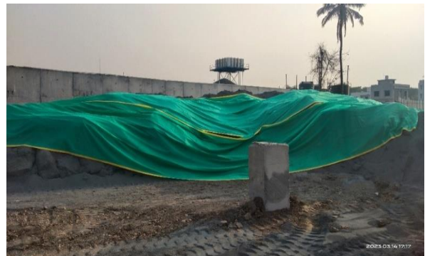
Covered the raw materials stacking in CY. 217
