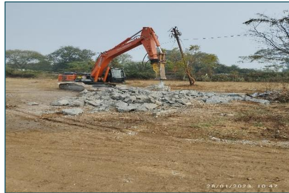
Pile head chipping work under progress and reuse in temporary road work, Converter in C6 Package
