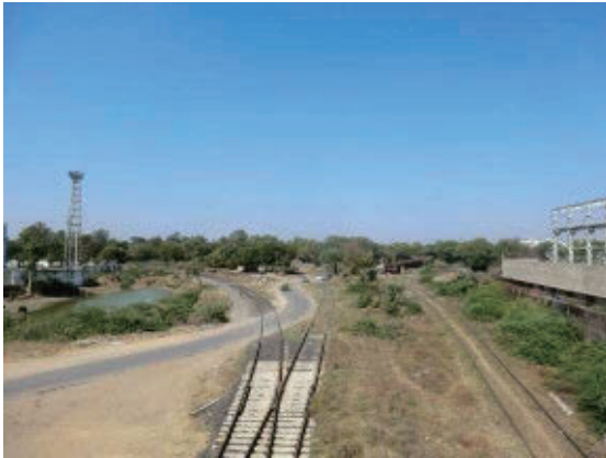
Figure 4.7-91 Entrance of Proposed Depot Location
