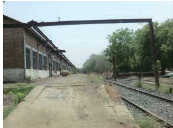
Figure 4.7-92 Warehouse for Rail Welding
