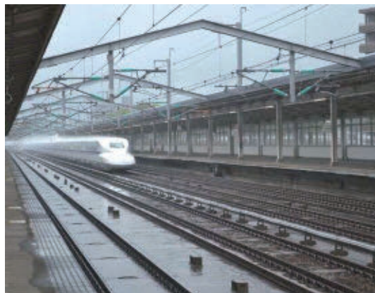
Figure 4.6-21 Slab Tracks of San-yo Shinkansen
