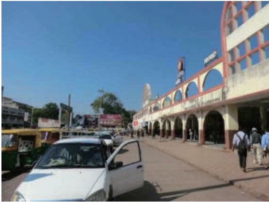
Figure 4.7-27 Anand Station Building and Plaza
