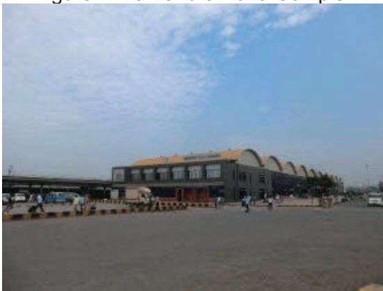
Figure 4.7-5 Lokmanya Station Building
