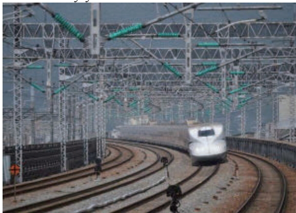
Figure 4.6-20 Ballast Tracks of San-yo Shinkansen
