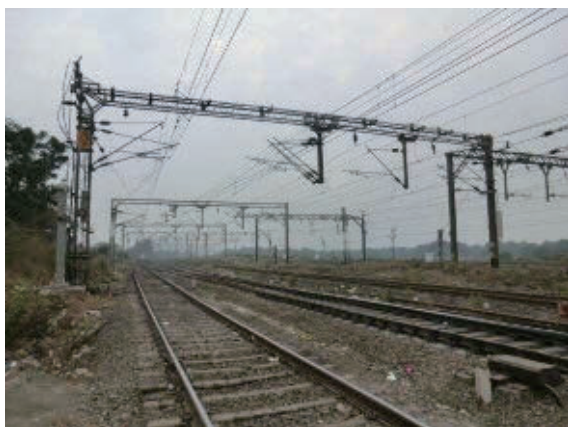
Figure 4.7-19 Existing Railway Line Near Proposed HSR Station
