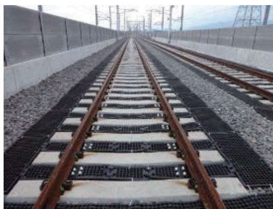
Figure 4.6-18 Ballast Track (installed with ballast screens)
