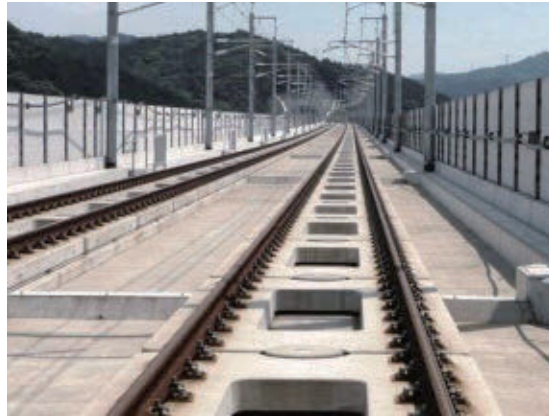
Figure 4.6-22 Frame-type Slab Track
