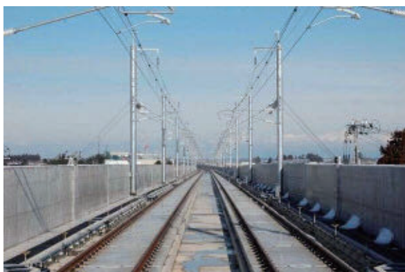
Figure 4.6-17 Plate-type Slab Track
