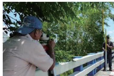
Figure 6.1-21 Vertical Control Survey (direct leveling)
