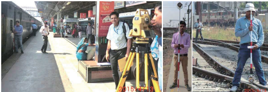
Figure 6.1-25 Topographic survey observation & Pole prism as target
