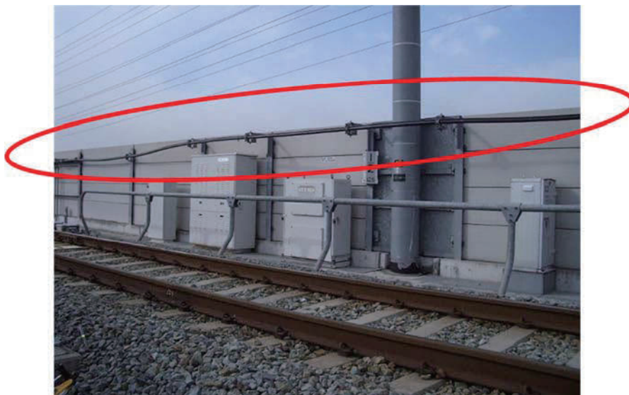
Figure 9.11-6 LCX Installation Example
