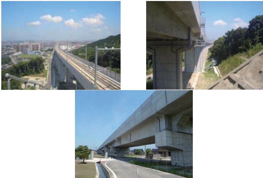
Source: Study Team, Source: http://www.pcken.or.jp Figure 9.3-1 Viaduct (PC T-shaped Girder)
