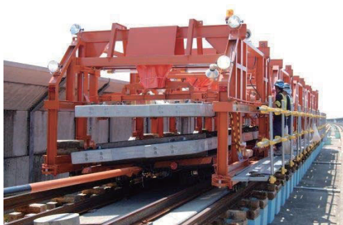
Figure 9.7-62 Lifting of Track Slabs
