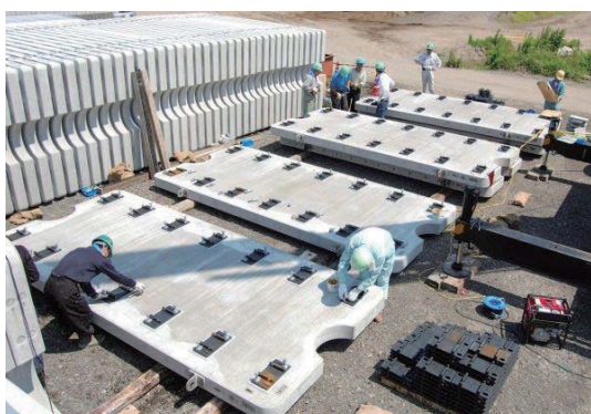
Figure 9.7-51 Fixing of Tie Plates
