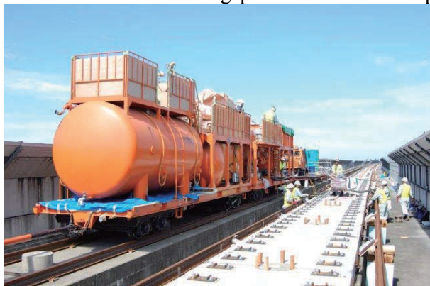
Figure 9.7-66 Injection of CA Mortar
