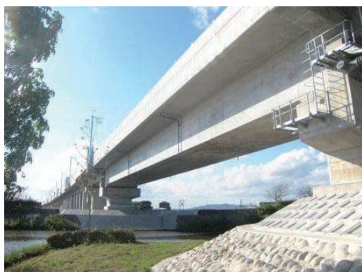
Figure 9.4-4 Bridge for Canal (PC Box Girder for River using Supporting)
