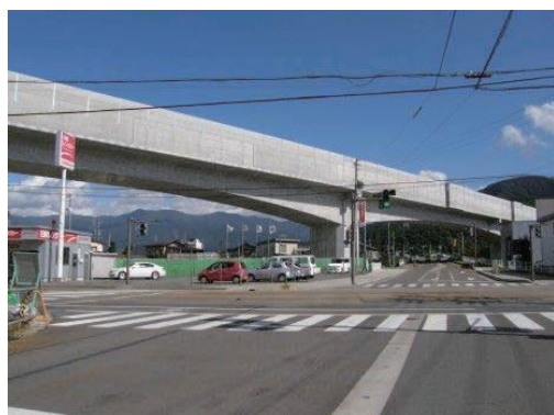
Figure 9.4-5 RUB (Continuous Bridge of PC – Box Girder using Cantilever Method)
