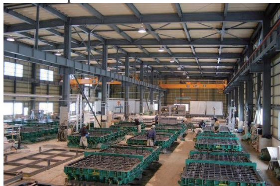
Figure 9.7-40 Track Slab Manufacturing Plant (Internal View)
