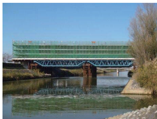
Figure 9.4-4 Bridge for Canal (PC Box Girder for River using Supporting)
