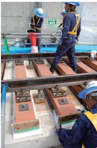
Figure 9.7-89 Injection of Resin
