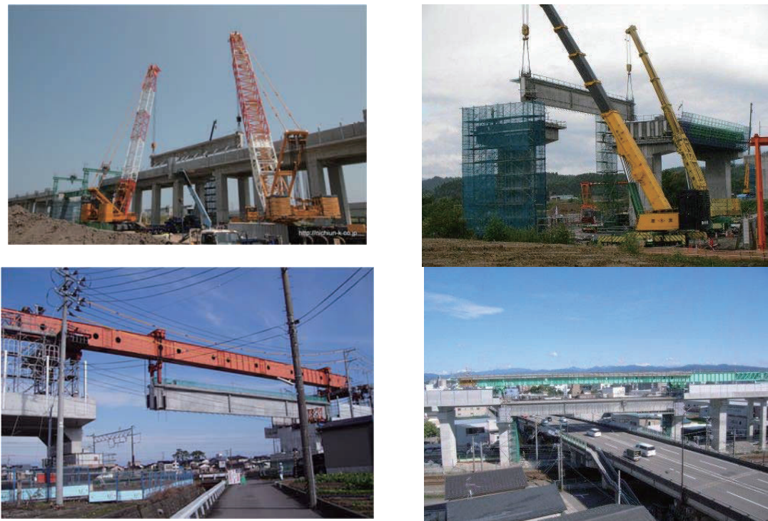
Source: http://www.pcken.or.jp Figure 9.3-2 Girder Erection (Crane / Erection Girder)
