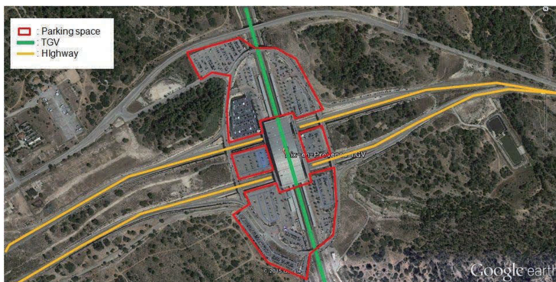
Figure 9.6-42 The Case of Aix en Provence Station of TGV, France
