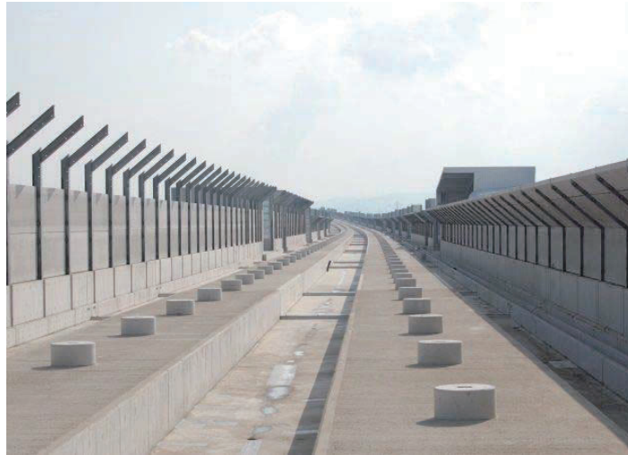
Figure 9.7-10 Completed Reinforced Concrete Track Bed
