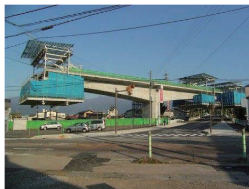
Figure 9.4-5 RUB (Continuous Bridge of PC – Box Girder using Cantilever Method)
