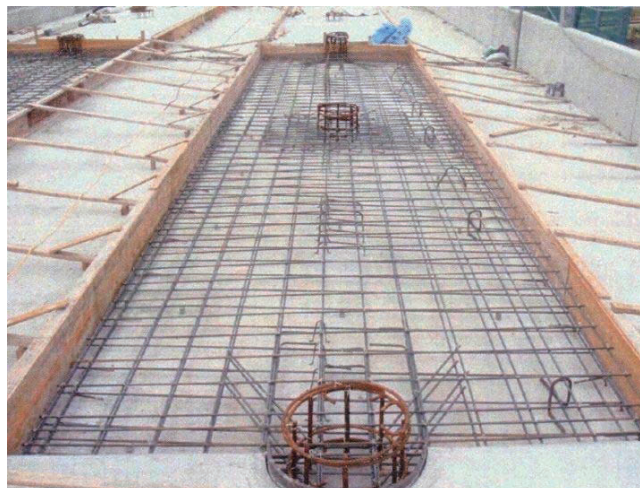
Figure 9.7-7 A scene of the Work to Construct a Reinforced Concrete Track Bed
