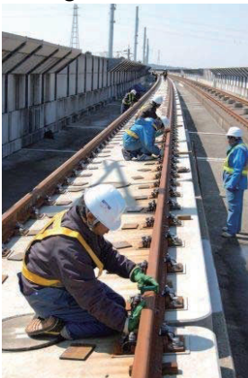
Figure 9.7-70 Adjusting of Rails
