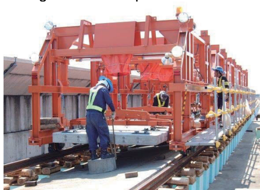
Figure 9.7-63 Laying of Track Slabs
