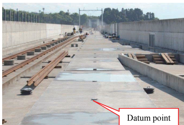
Figure 9.7-17 Reinforced Concrete Track Bed at Turnout
