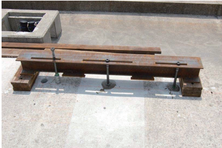
Figure 9.7-86 Planting of Steel Bar Insert
