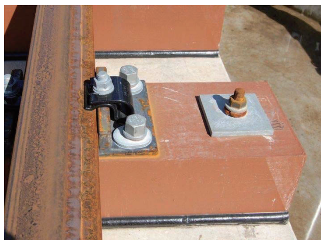
Figure 9.7-90 Fastening of Sleeper
