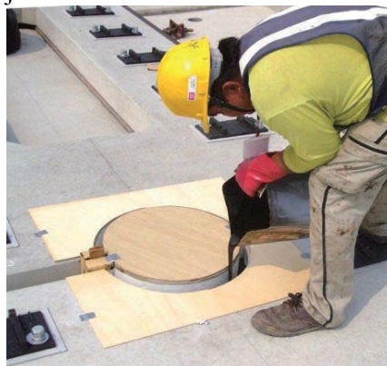
Figure 9.7-67 Injection of Urethane Resin around the Concrete Projection
