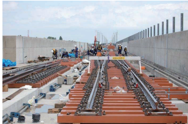
Figure 9.7-88 Fabrication of Turnout
