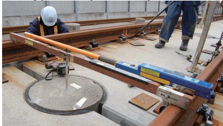
Figure 9.7-70 Adjusting of Rails
