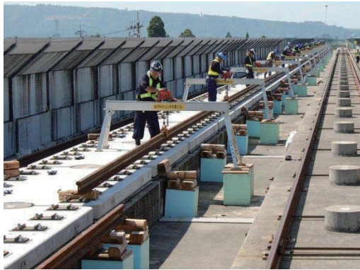
Figure 9.7-68 Relocation of Rails
