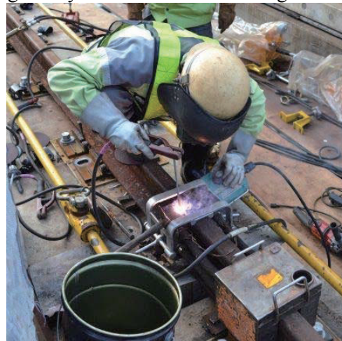
Figure 9.7-76 Tertiary Welding
