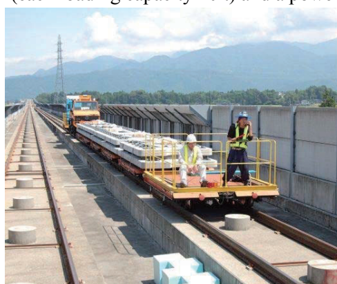
Figure 9.7-59 Transport of Track Slabs
