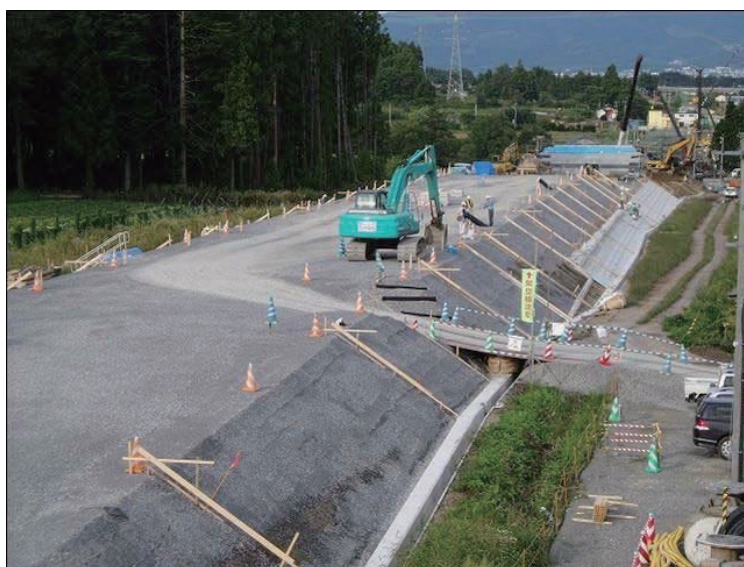
Figure9.2-12 Japanese Experience of the Reinforced Embankment Structure
