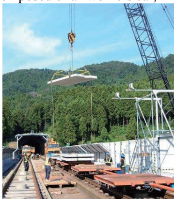
Figure 9.7-58 Loading the Train with Track Slabs
