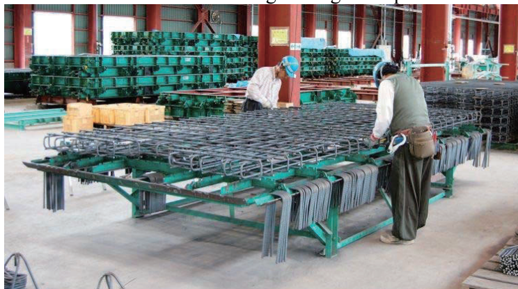
Figure 9.7-42 Fabrication of a Reinforcing Bar Cage
