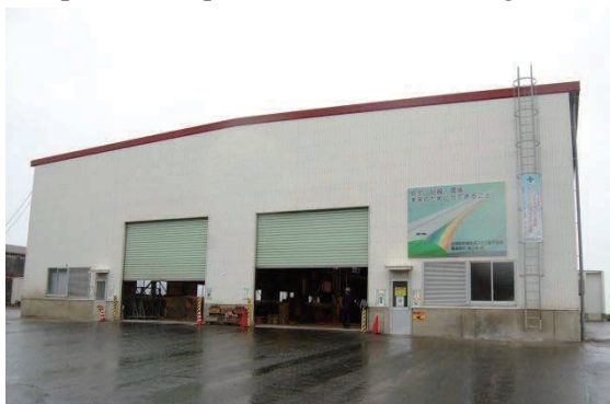
Figure 9.7-39 Track Slab Manufacturing Plant (External View)
