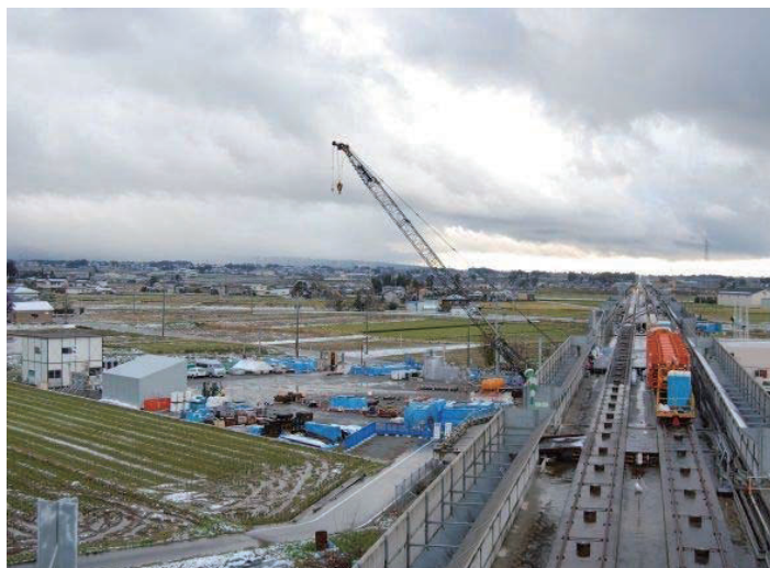
Figure 9.7-35 Track Construction Work Base
