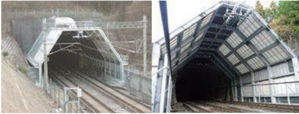
Figure 5.2.11: Examples of Tunnel Boom Insulation
