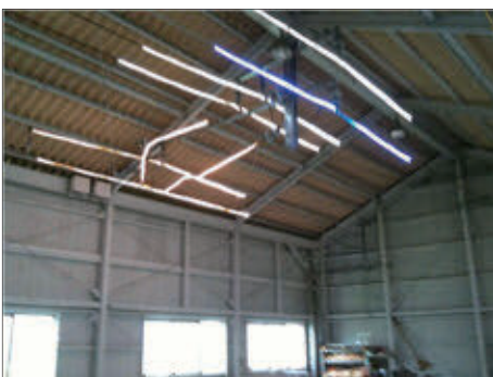
• Position to the overhead wire
