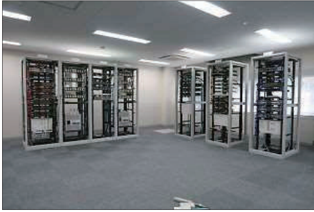
• Telecommunication training room
