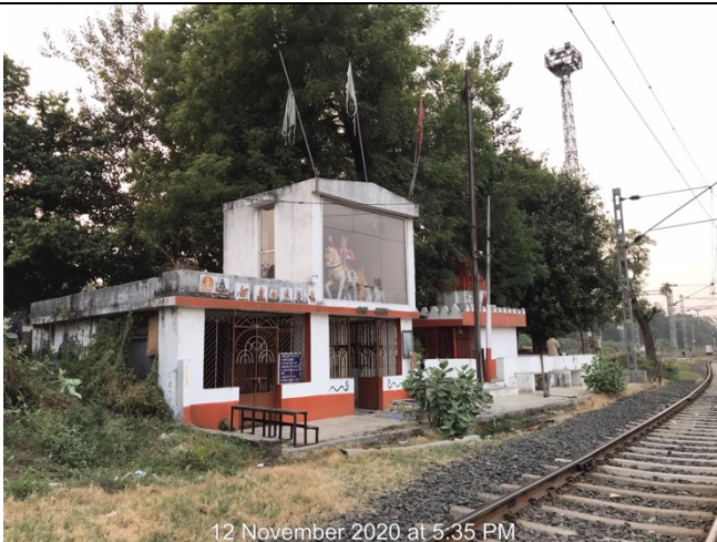
Temple being impacted (Before Dismantling) in Railway Yard (Vadodara District)
