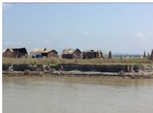
Erosion of the Char Land
