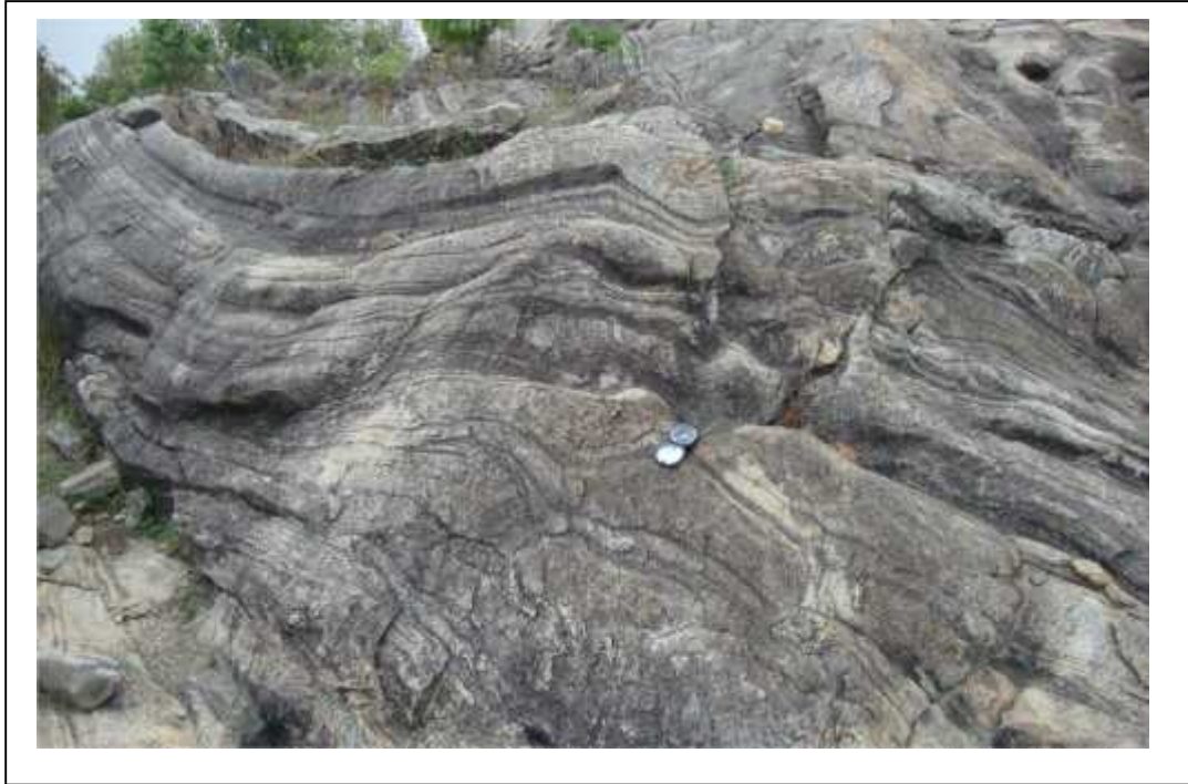
Hard and competent quartzo-feldspathic gneiss exposed on the left abutment of the proposed upper dam alignment of Turga PSP. The bedrock also shows broad warping.
