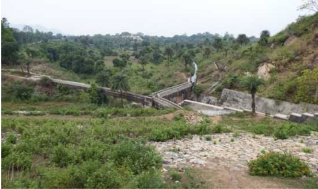
Plate-9.5 : D/s of Existing Irrigation Dam, Pathardih
