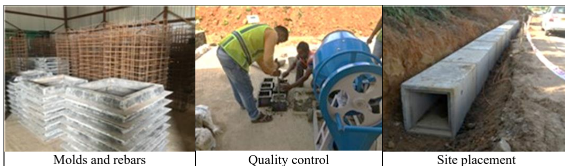
Figure 3-15: Precast method Adopted for the Construction of NH44
