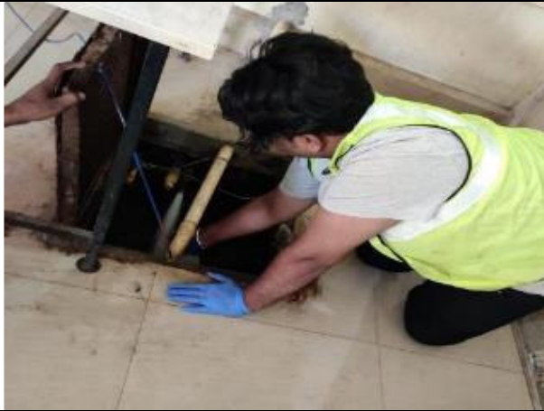
GW2- Bore Well near Marathahalli, Outer Ring Road
