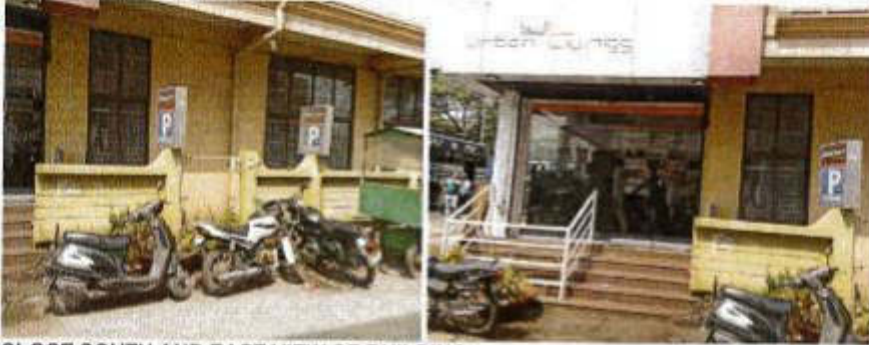
CLOSE SOUTH AND EAST VIEW OF BUILDING
