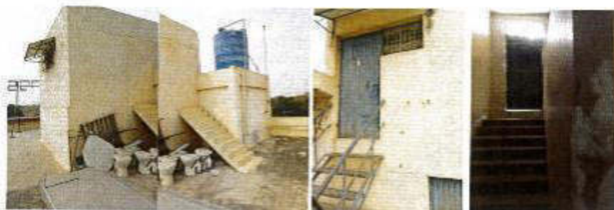
NORTH AND SOUTH VIEW OF STAIRCASE AND LIFTMACHINE ROOM
