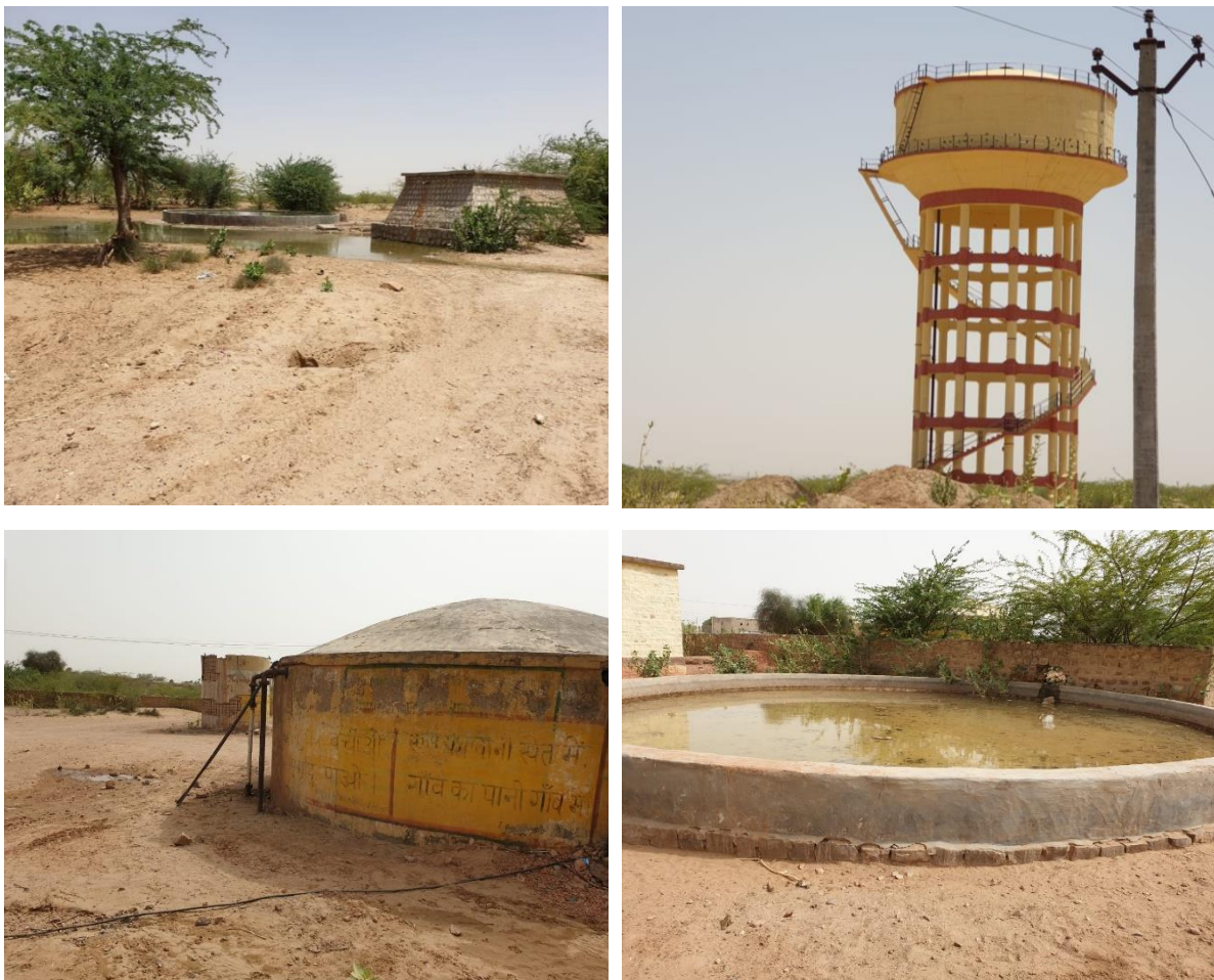
Water Facility in Harwa Village
