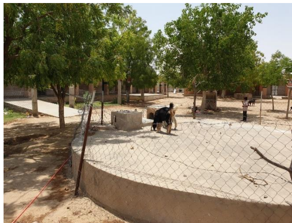
Drinking Water Facility at Reevadi School
