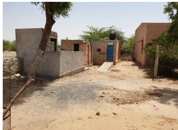
Toilet Facility at Reevadi School
