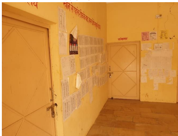
Community Center at Reevadi
