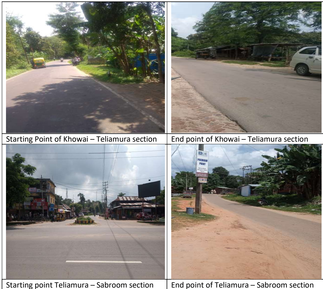
Figure 1.2: Photographs showing starting and end points of the project alignment
