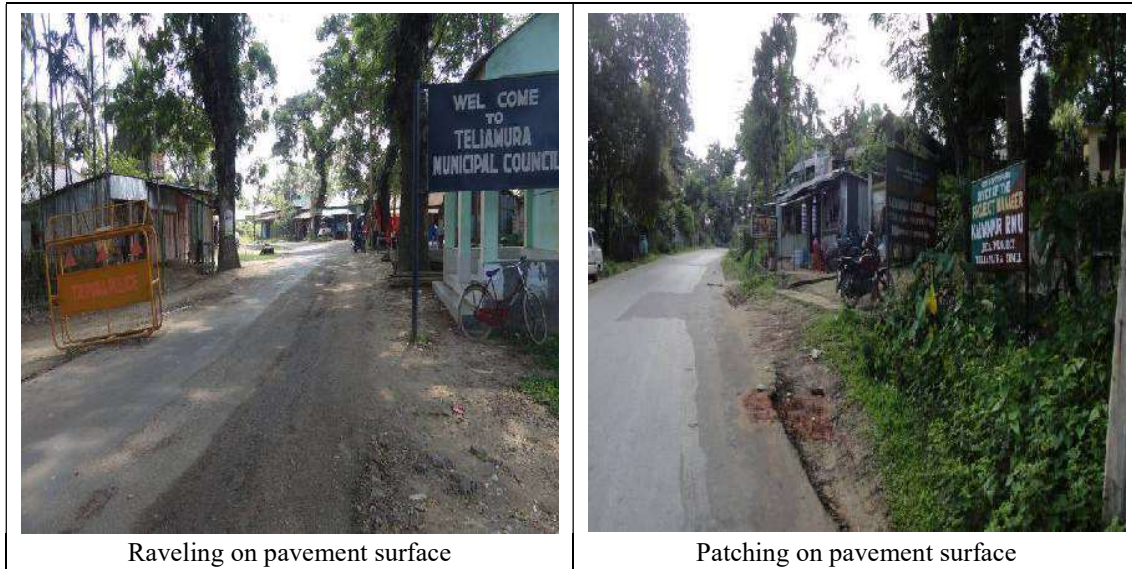
Figure 5-24: Pavement Conditions
