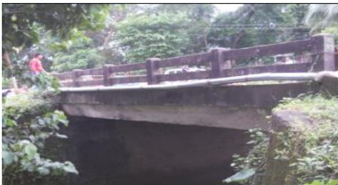
Figure 8: image of existing minor bridge at chainage 18+015km
