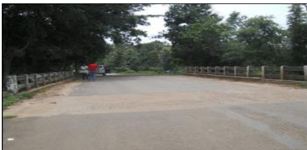
Figure 7: image of existing major bridge at chainage 12+400km
