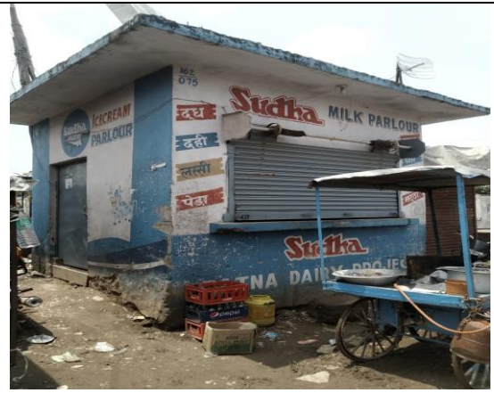
MT1 – Affected structure of Mithapur station
