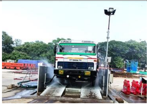
Wheel washing facility
