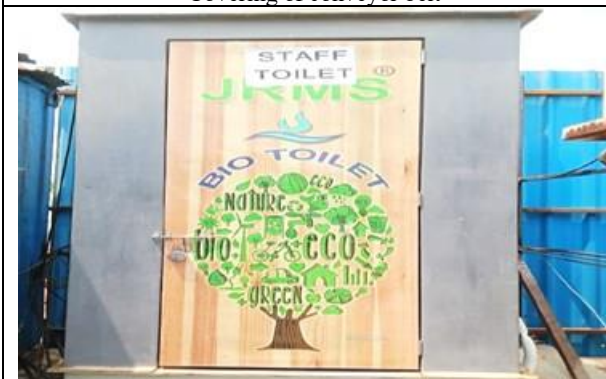
Use of bio toilet at site
