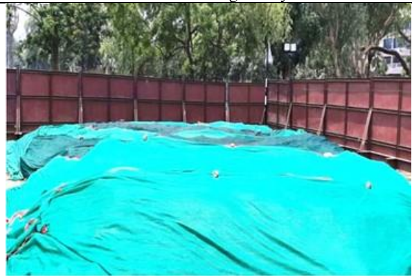
Covering of dry soil/sand at site
