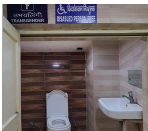
Multi and Transgender toilet
