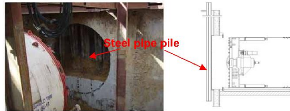
Case1 (Launching: Used Steel Pipe Pile)
