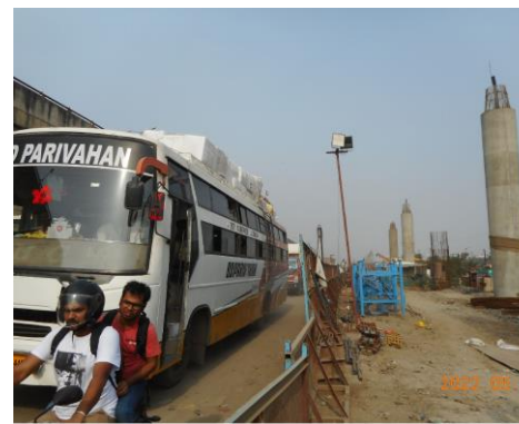
Corridor2 ST11 Zero Mile
