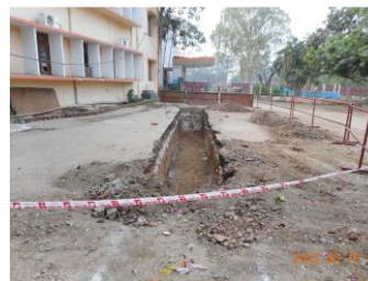
Figure 5-34: Construction Condition of Guide Wall for Diaphragm Wall Construction at Corridor2 ST05 Moin UI Haq
