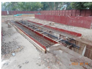
Figure 5-34: Construction Condition of Guide Wall for Diaphragm Wall Construction at Corridor2 ST05 Moin UI Haq
