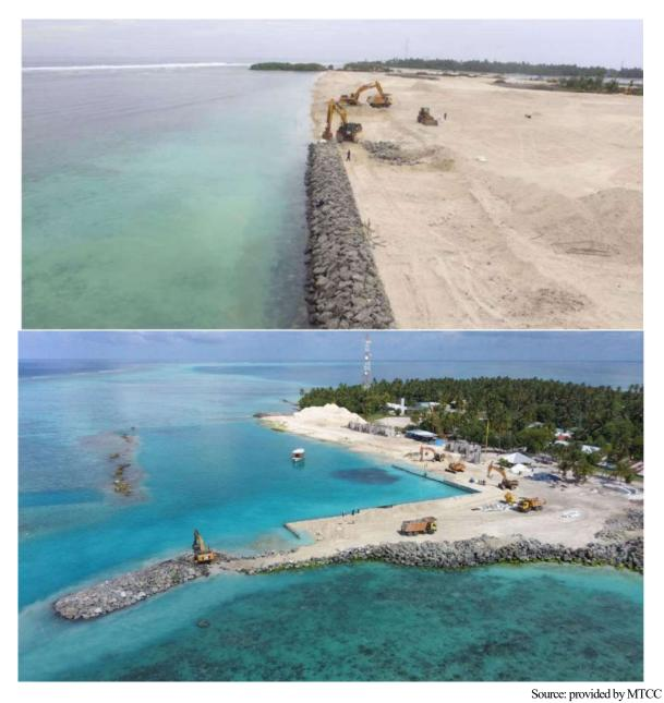
Figure 5.8.32 Installation of the Jetty and Revetment
