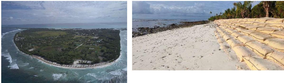
**Figure 4.2.7 Sandbag Revetment under Construction by MNPFI as an Emergency Project (as of September 2022)**
