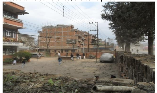
Photo 4. Road-side use by local school as play-ground and electric poles & transformers
