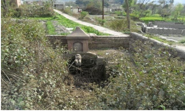
Photo 9. Non-functioning Dunge Dhara along Road
