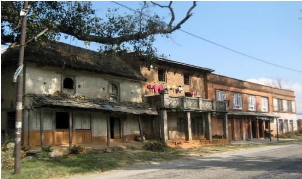
Photo 5. Some very old houses along Road, some newer house, need to be removed
