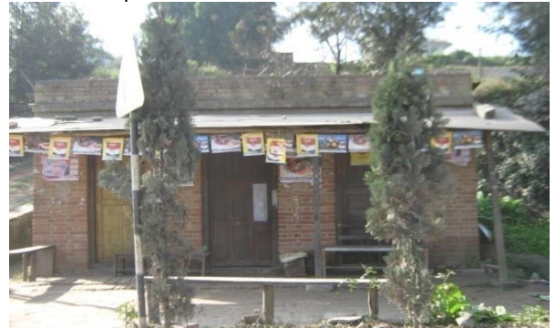
Road 6. Sheds along Road, used for small shops, need to be removed
