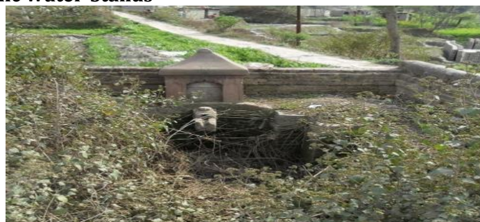
Figure 5.3-2 Non Functioning Small Water Sprout
