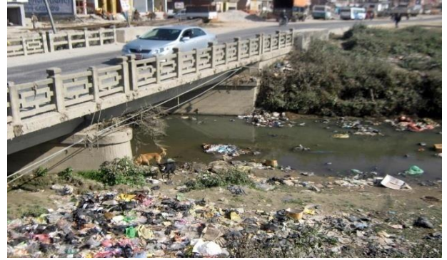
Photo 10. Low free-board at Banena Bridge during dry season, overflow during monsoon
