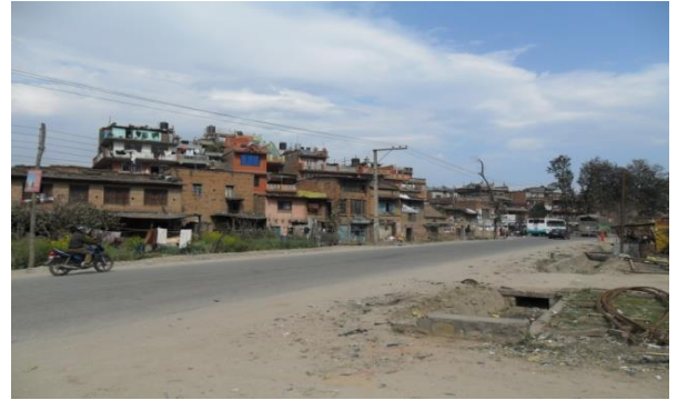
Photo 2. Road-side houses near Jagati, total 13 nos. old houses to be demolished, & electric poles
