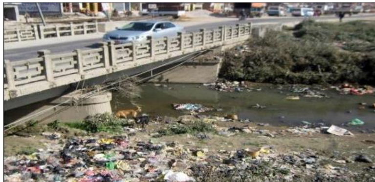
Figure 5.1-1 High Water Flow Level at Punyamati Khola Bridge Site
