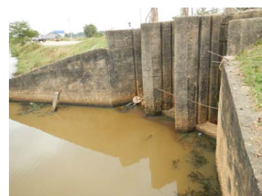
Intake of Ka Ek Tom Reservoir (View from Upstream)
