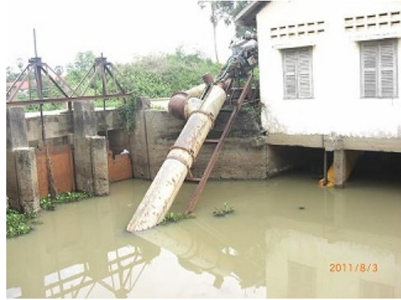
Existing intake and pump station at Tonle Bati Lake (intake gates are heavily deteriorated and pump capacity is much less than required one)
