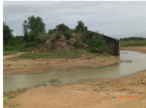
Slakou river and Breached Dike of Tumnup Lok Reservoir
