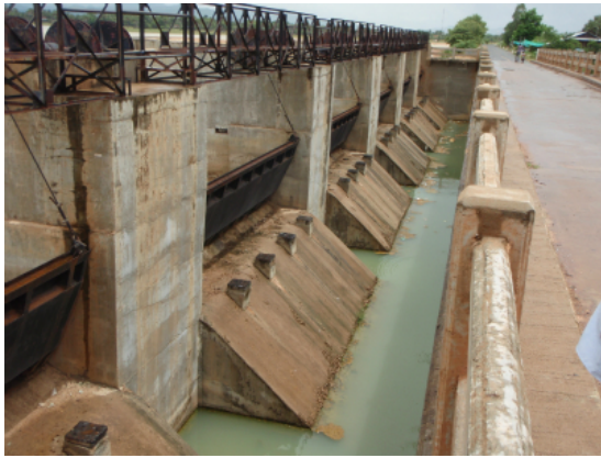
Spillway of Kpob Trobek Reservoir
