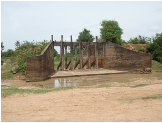
Intake gate on Tumnap Lok Reservoir
