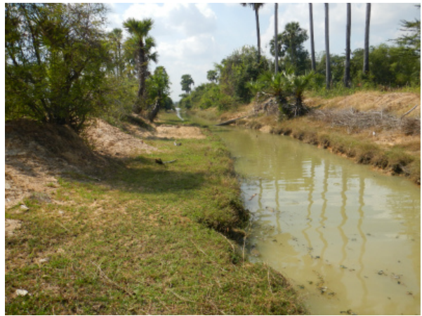
Main Canal 35 (near Khpob Krous Reservoir)
