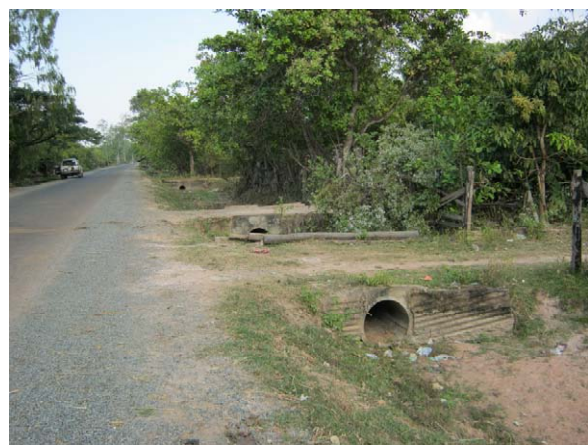
Pipe culvert on main canal (to be replaced)
