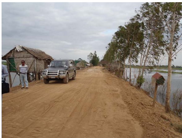
Srass Prambai Reservoir Dike (already rehabilitated)
