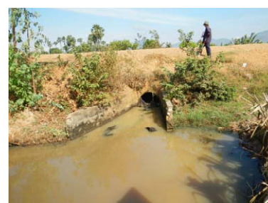
Culvert of O Kbear Reservoir (View from Downstream)
