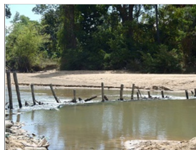
Existing Temporary Headworks
