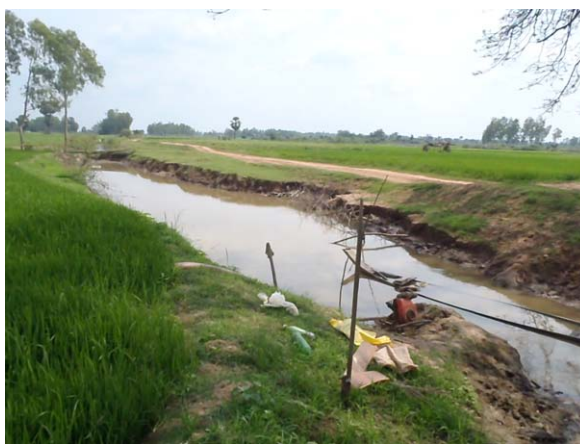
Main canal after recession
