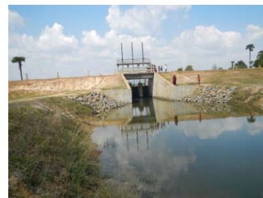
Intake of Khpob Krous Reservoir (View from Downstream)
