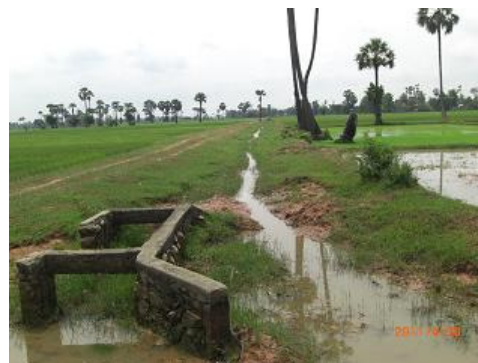
Canal 24 and Deteriorated Division Structure
