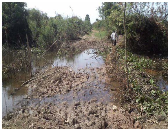
Srass Prambai Reservoir Dike (to be rehabilitated)
