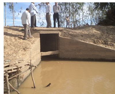
Existing Intake Culvert
