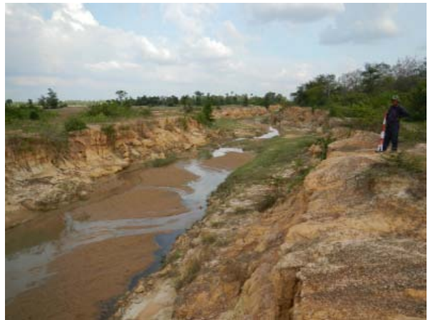
Main Canal 35 (Downstream area)
