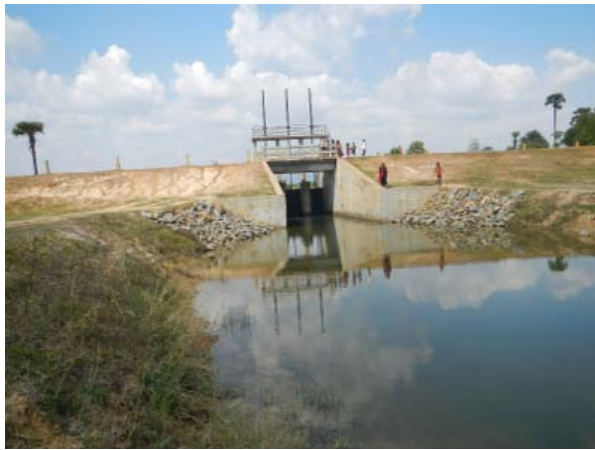
Intake of Khpob Krous Reservoir
