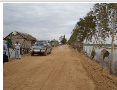
Dike of Srass Prambai Reservoir
