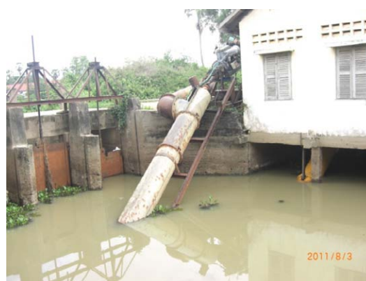
Intake and Pump Station at Lake Tonle Bati
