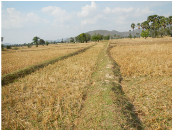
Main Canal 35 (3 km downstream of Khpob Krous Reservoir)
