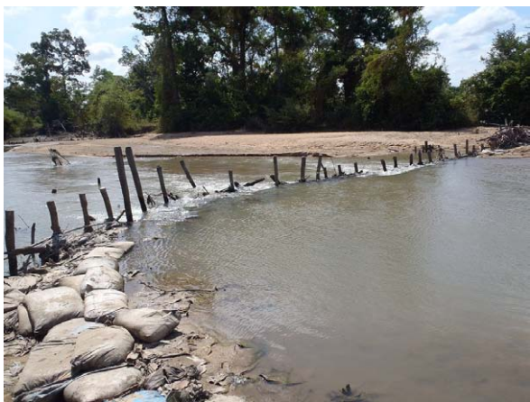
Temporary weir for Daun Pue Intake made with sand bags and wooden material
