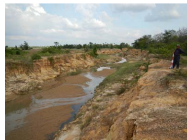
Main Canal 35 (Downstream of Kokir River Confluence)
