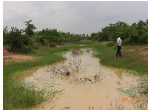
Canal condition of the Diversion Canal
