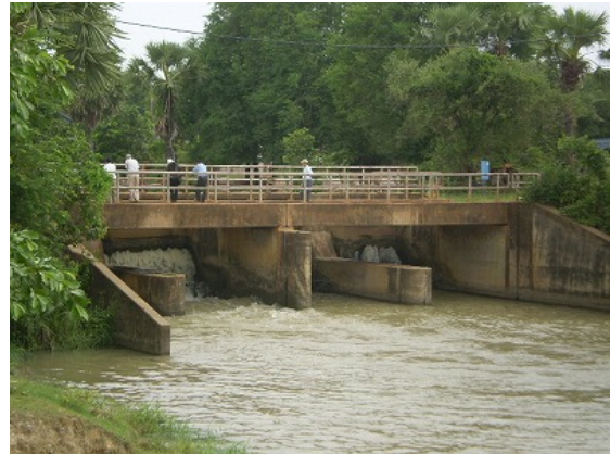
Andong Sla Intake (downstream view)
