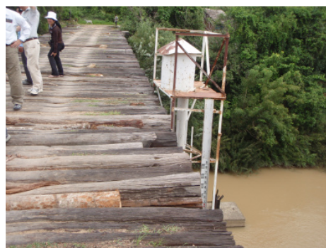
Water Gauging Station at Peam Khley
