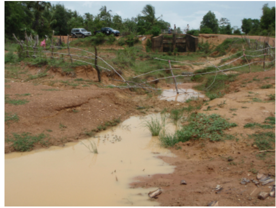
Diversion structure on Tumnap Lok Reservoir
