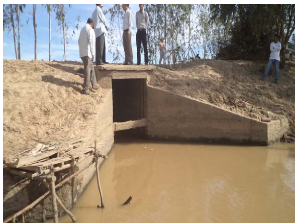
Intake culvert on reservoir dike
