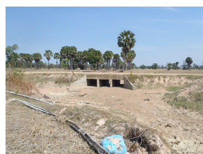
Existing Main Canal and Culvert
