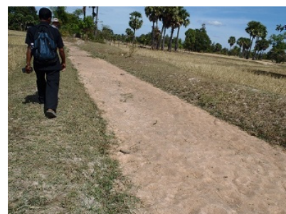
Existing Secondary Canal
