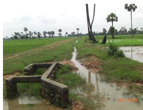
Canal 24 and Deteriorated Division Structure
