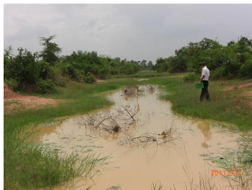
Canal Condition of the Diversion Canal
