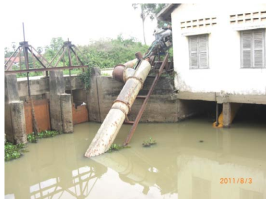
Intake and Pump Station at Lake Tonle Bati
