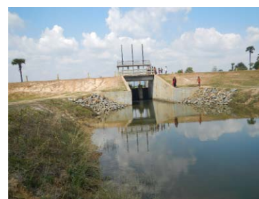
Intake of Khpob Krous Reservoir (Downstream View)
