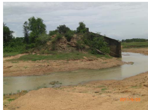
Slakou River and Breached Dike of Tumnap Reservoir
