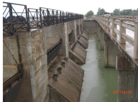
Gated Spillway and Bridge on Kpob Trobek Reservoir
