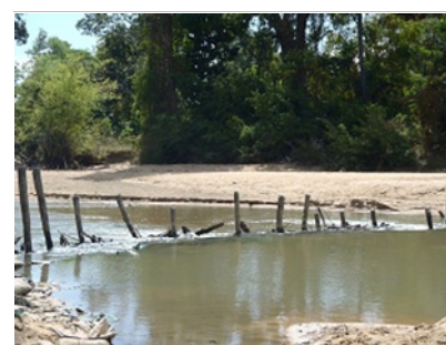
Existing Temporary Headworks
