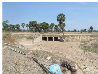
Existing Main Canal and Culvert
