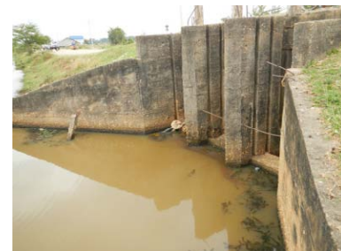
Intake of Ka Ek Tom Reservoir (Upstream View)
