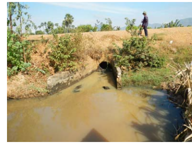
Culvert of O Kbear Reservoir (Downstream View)
