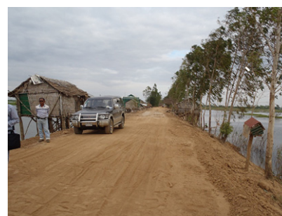
Existing Srrass Prambai Reservoir Dike (Rehabilitated Section)
