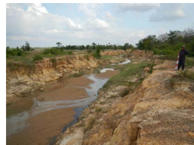
Main Canal 35 (Downstream of Kokir River Confluence)
