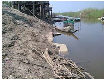
Photo View from Downstream
