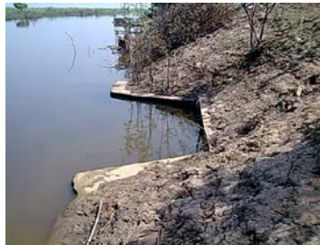
Photo View from Downstream
