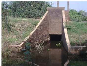
Photo View from Downstream
