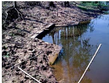
Photo View from Downstream
