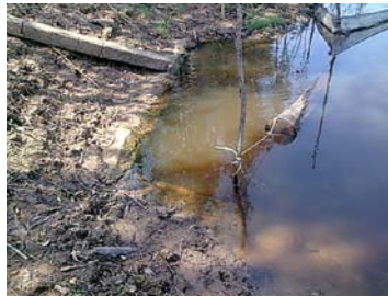
Photo View from Downstream
