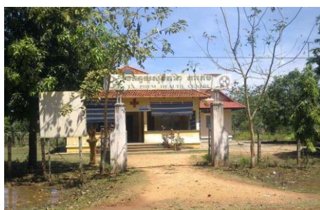
Steel fence and entrance gate of Ta Phem Commune Health Center in COI of SC 3D of Original and Proposed Plan
