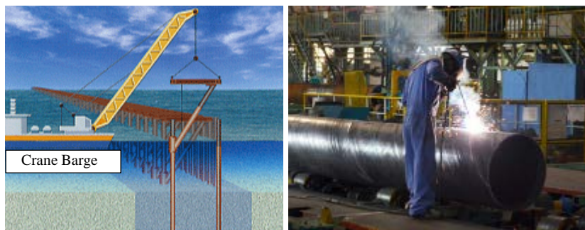
Figure 1.46. Construction of Berth Section in Parallel
