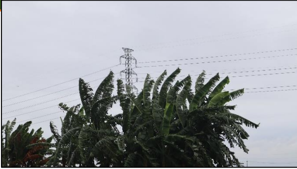
sta 20+663,087 (Desa Tanjung Rasa, Kecamatan Tambak Dahan STA 20+663,087 (Tanjung Rasa Village, Tambak Dahan District
