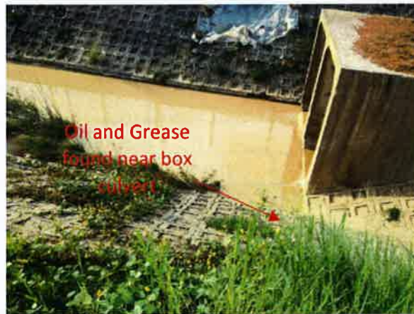
Figure 2 Found oil and grease around the box culvert (But cannot see in photo because of the thin layer of oil is dispersed on water)
