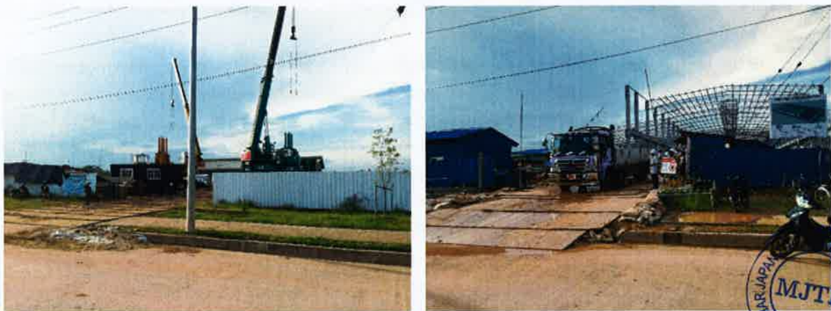
Figure 3 Construction Site near around the box culvert
