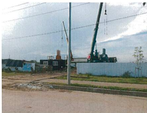
Figure 2 Construction Site near around the box culvert
