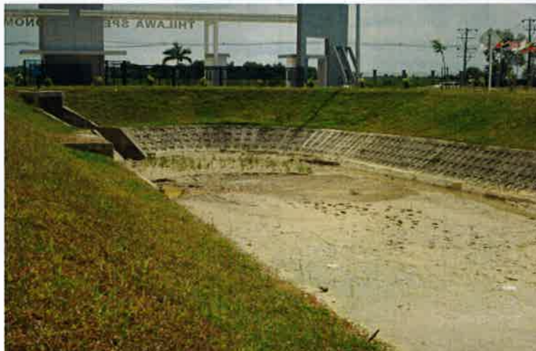
Figure 8. Condition of SW-5 and its surrounding
