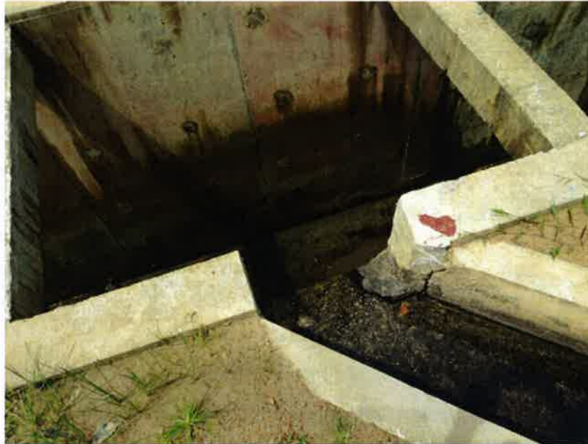
Figure 9. Condition of SW-6 and its surrounding
