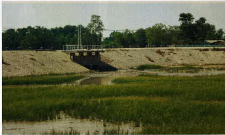
Figure 7. Condition of SW-1 and its surrounding
