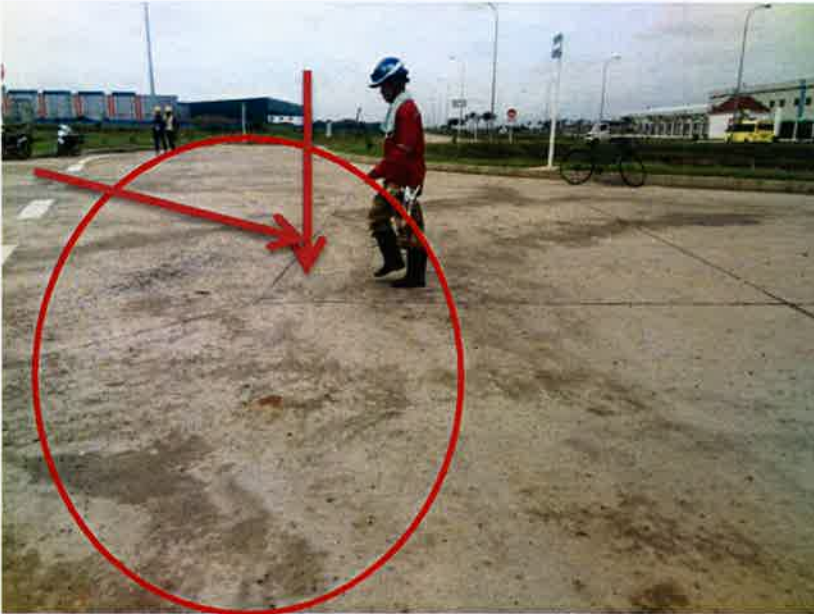
Cleaning work for broken glass
