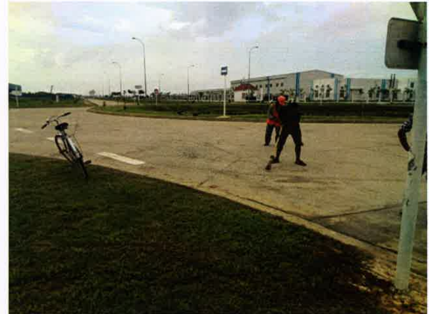
Cleaning work for broken glass
