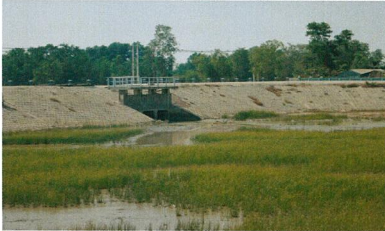
Figure 7. Condition of SW-1 and its surrounding
