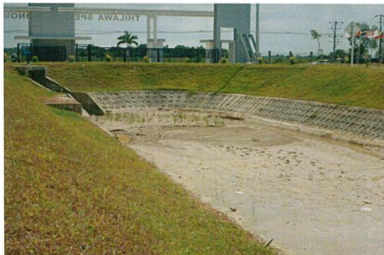
Figure 8. Condition of SW-5 and its surrounding
