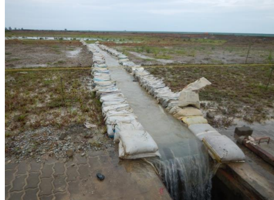
Tentative Drainage (to prevent soil erosion)
