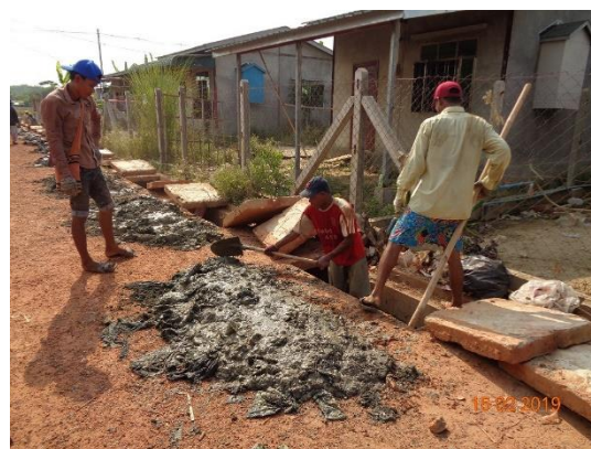
Photo 7-4 Drainage Cleaning
