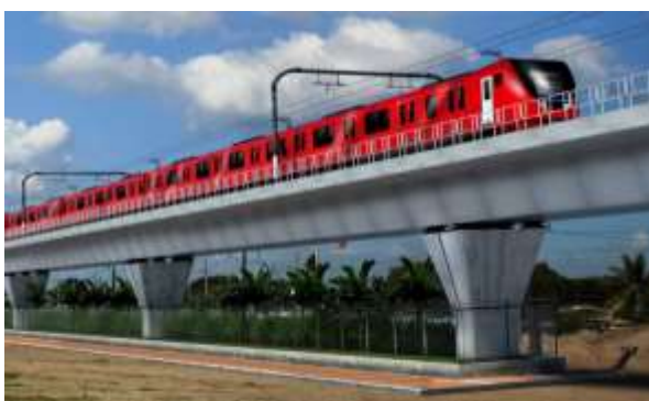
Figure 4.2.1 PC Segmental Box Girder
