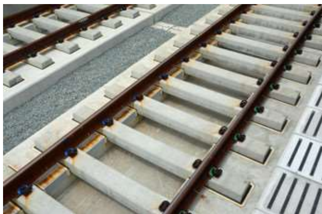
Figure 4.2.70 Ballast less Track structure (elastic sleeper directory fastened track on concrete bed)
