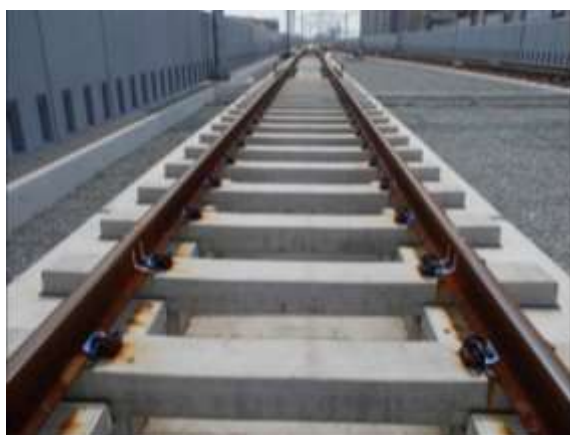
(iii) Elastic Sleeper Directly Fastened Track
