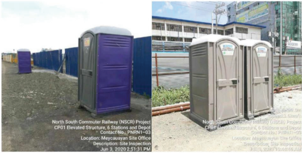
Portalets deployed at Meycauayan NSCR alignment works.
