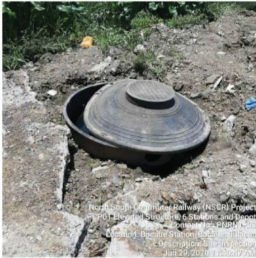
On-going installation and assembly of underground septic tank for temporary toilet at Bocaue construction site.
