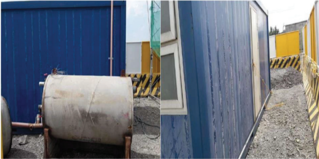
Temporary toilet facility at Malanday Depot with fabricated septic tank.
