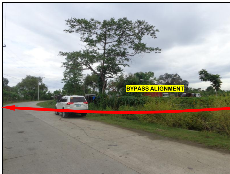
Photo No. 1.1.1-12 Bypass alignment intersecting the Malagamot Road in Brgy. Indangan, between Sta. 28+700-28+800 .
