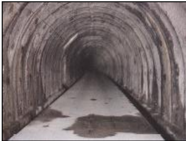
Photo No. 7.2.2-1 Evacuation tunnel exit. (Source JICA Study Team, July 2014)
