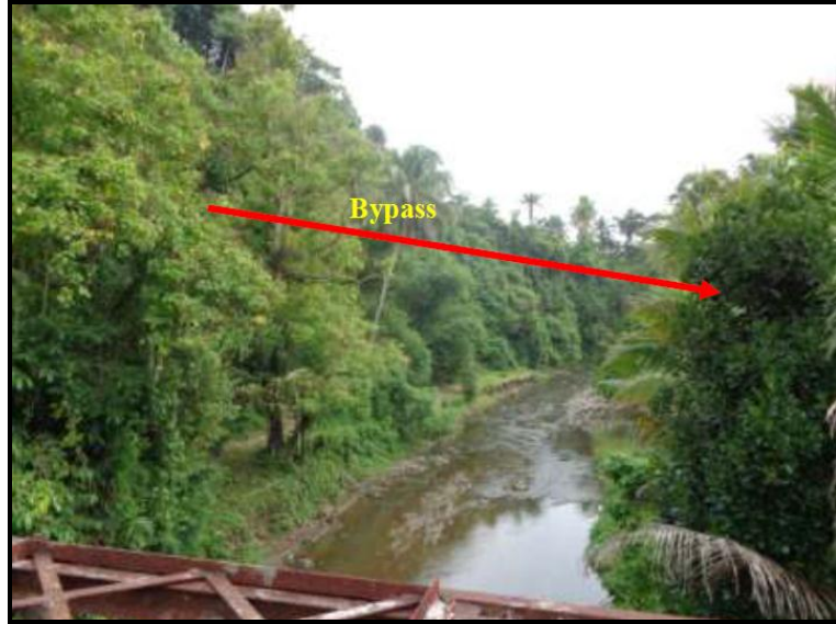
Photo No. 1.3.2-1 Photo showing the west side of the area to be traversed by the proposed tunnel.
