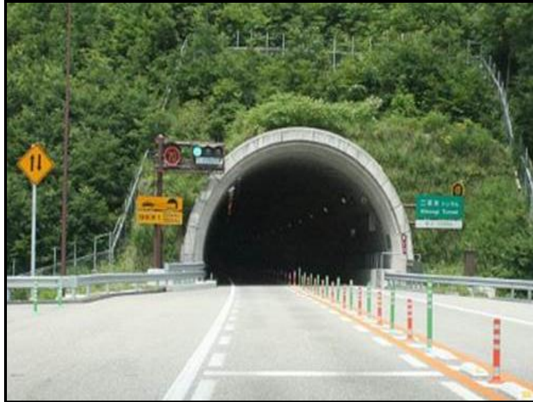
Photo No. 1.4.2-1 Photo showing the portal of a 2-lane tunnel in Japan. (Source: JICA Study Team, July 2014)
