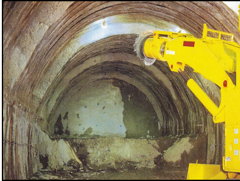
Photo No. 1.5.3-3 Photo showing excavation by a Road Header (Source: JICA Study Team, July 2014)
