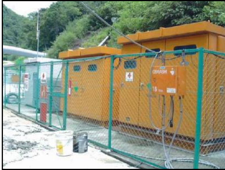
Photo No. 1.5.3-5 Electric Power Station and Receiving Box (Source: JICA Study Team, July 2014)
