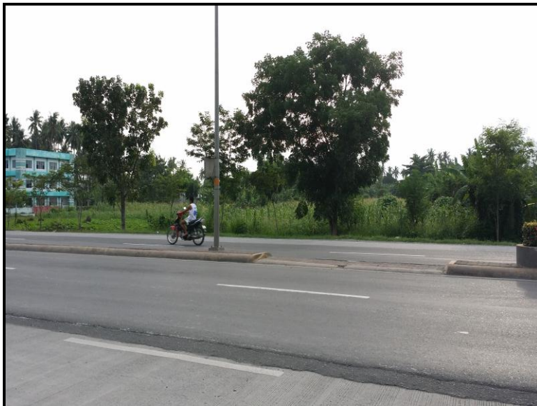
Photo No. 1.1.1-28 General view at the terminus of the proposed bypass alignment along the Davao-Agusan National Highway in Brgy. J.P. Laurel, Panabo City.
