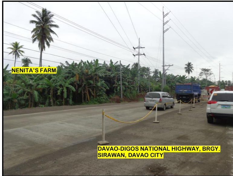
Photo No. 1.1.1-1 Taken at the start of the proposed Davao City Bypass Construction Project alignment, Sta. 0+000 along the Davao-Digos National Highway in Brgy. Sirawan, Davao City.
