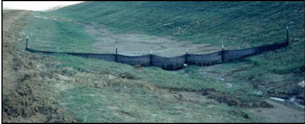
Photo No. 6 Silt fence to mitigate downward mobilization of loose earth materials during construction works.
