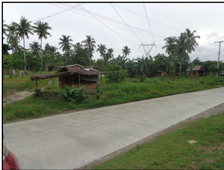
Photo No. 1.1.1-14 Photo of the taken at the intersection of the bypass alignment and Buhangin Road in Brgy. Mahayag between Sta. 38+300-38+400 .
