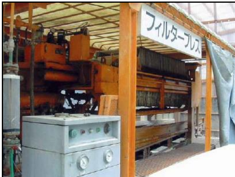
Photo No. 1.5.3-8 Dust Water Filter Equipment (Source: JICA Study Team, July 2014)
