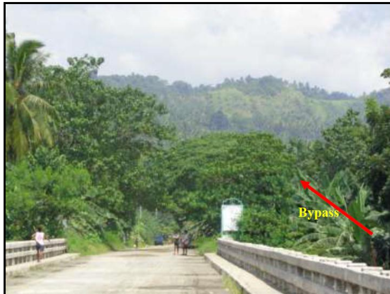
Photo No. 1.3.2-2 Taken at the east side section of the tunnel.
