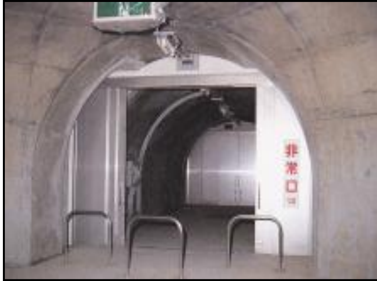
Photo No. 7.2.2-2 Evacuation tunnel exit. (Source JICA Study Team, July 2014)
