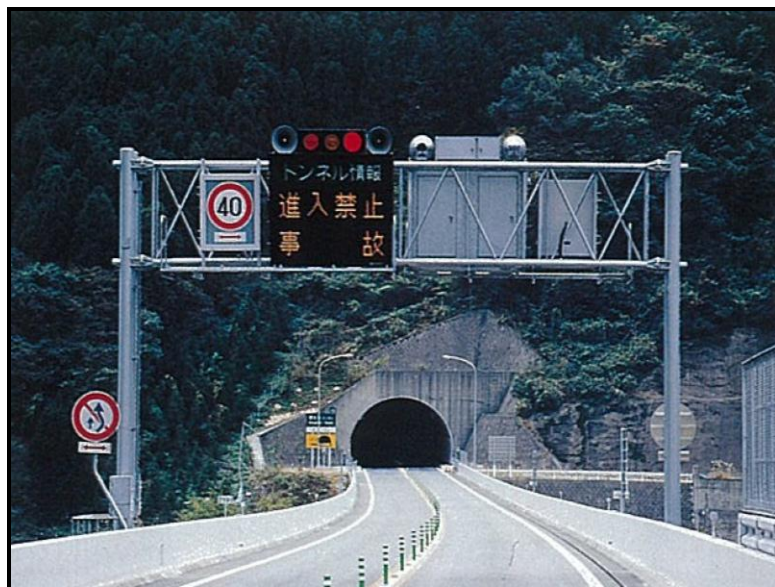
Photo No. 1.4.2-3 Variable Information signboard (Type D). (Source JICA Study Team, July 2014)
