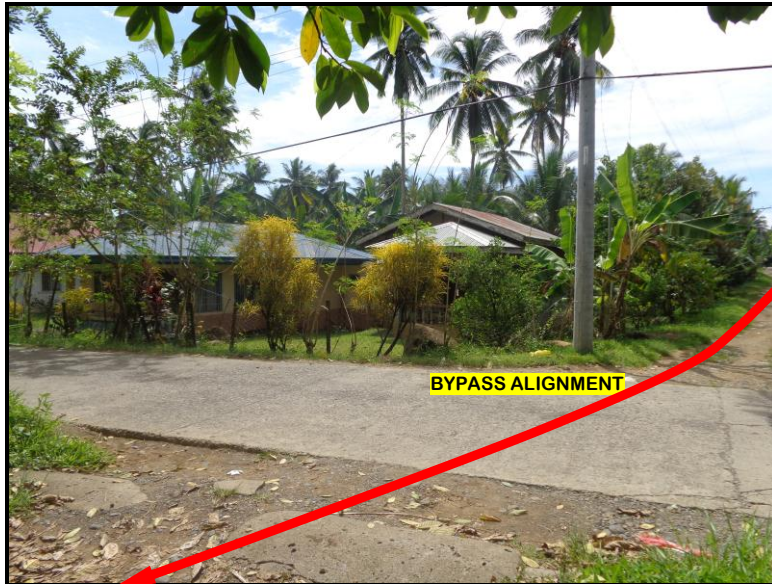
Photo No. 1.1.1-5 Some residential structures likely to be affected by the proposed bypass alignment along U.P. Road in Brgy. Mintal ( Sta. 9+600-9+700 ).
