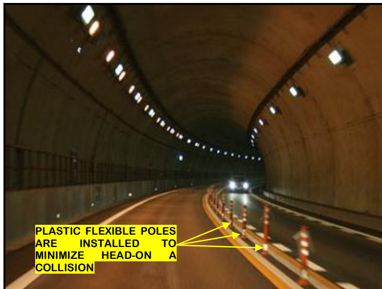
Photo No. 1.4.2-2 Photo showing the well-lighted interior of a 2-lane tunnel in Japan. Notice the plastic (flexible) poles installed at the center of the roadway which serve as dividers to minimize a head-on collision. (Source: JICA Study Team, July 2014)
