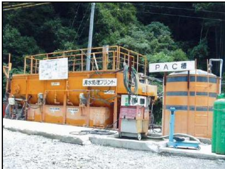
Photo No. 1.5.3-6 Sewerage Facilities (Source: JICA Study Team, July 2014)
