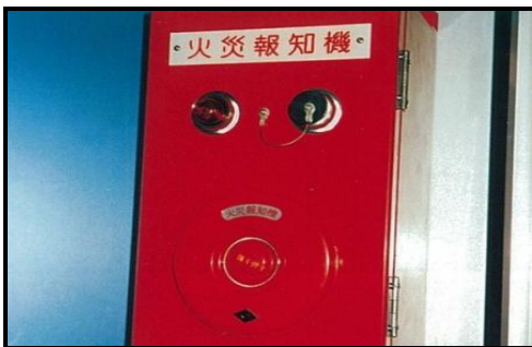
Push-Button Notification Equipment
