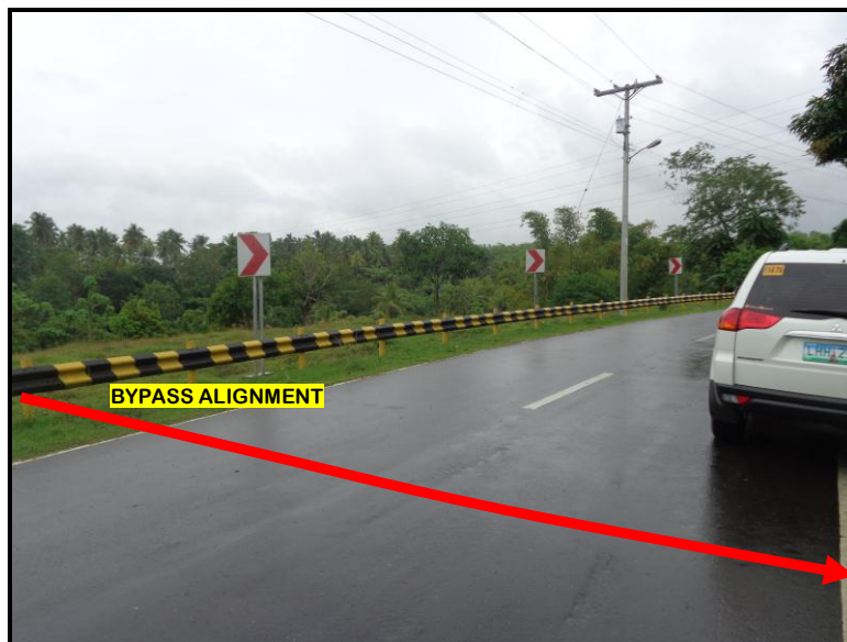
Photo No. 1.1.1-2 The proposed bypass alignment will intersect the existing Bayabas-Eden Road in Brgy. Marapangi, Davao City between Sta. 2+800-2+900 .
