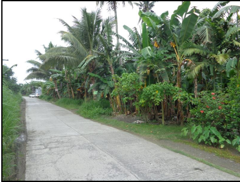
Photo No. 1.1.1-17 Photo of the taken at the vicinity of the proposed bypass alignment crossing an existing road in Brgy. Lasang at Sta. 44+000 .
