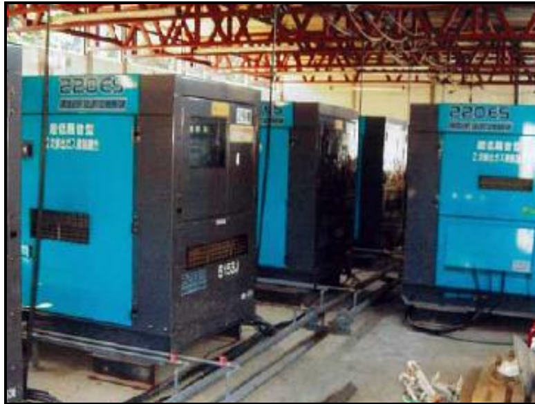
Photo No. 1.5.3-7 Generator Room for Tunnel Construction (Source: JICA Study Team, July 2014)
