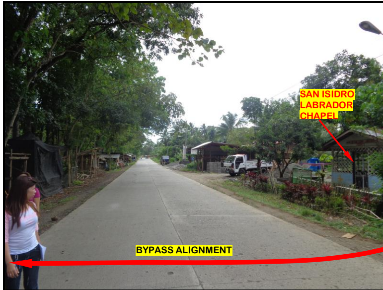
Photo No. 1.1.1-7 Taken at the intersection of the proposed bypass alignment and Mintal Road, between Sta. 12+900-13+000 in Brgy. Mintal.
