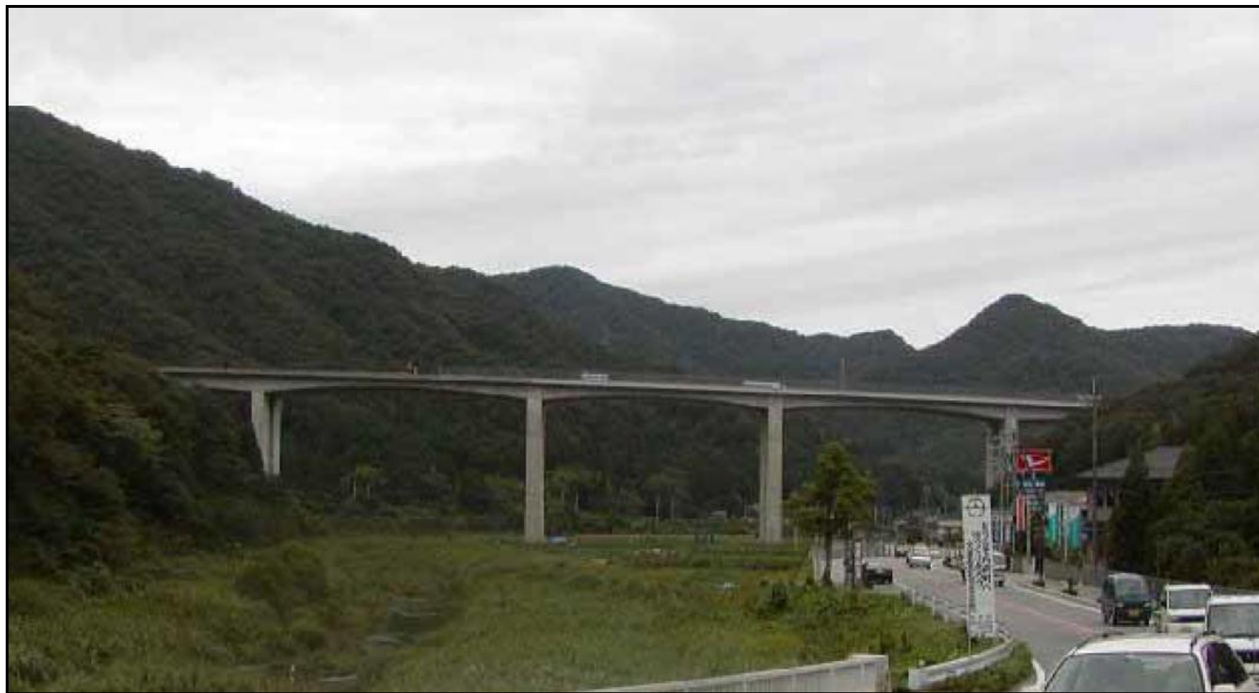
Figure 1.4.3-11 Photo Showing a Typical Cantilever PC- Box Concrete Structure Type
