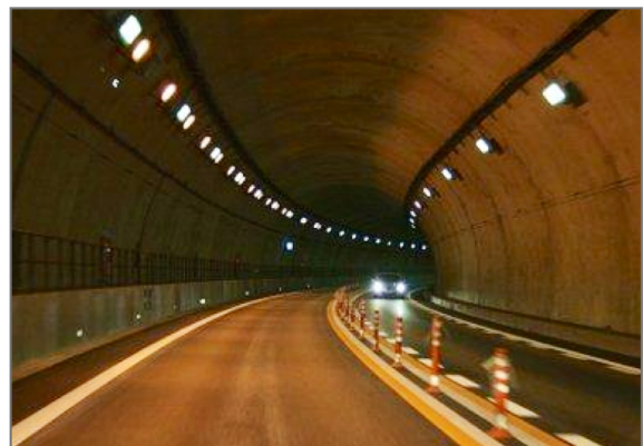
1-7 (c) Well-lighted interior of a 2-lane tunnel in Japan. Plastic (flexible) poles are installed at the center of the roadway for safety. Source: JICA Study Team 2014
