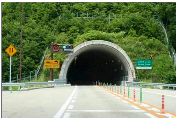
1-7 (b) Portal of similar 2-lane tunnel in Japan. Source: JICA Study Team 2014
