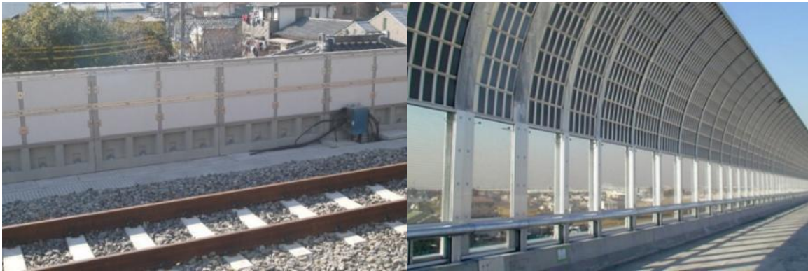
Figure 56. Noise Barrier (noise reduction ~5dB)
