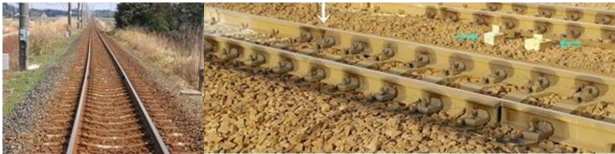
Figure 57. Long Welded Rail and Expansion Joint
