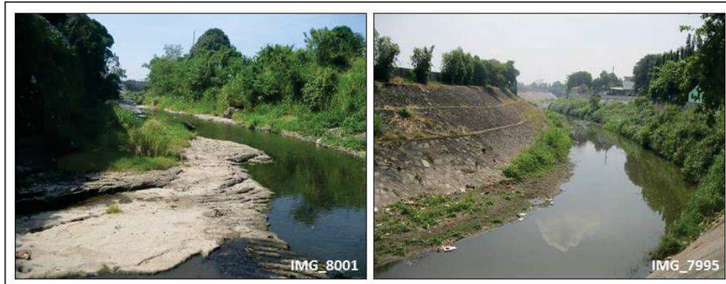
Figure 4.10: Exposure of tuffaceous sandstone along the Ylang Ylang River Improvement Project (left photo). Deep river valley along the Rio Grande River Improvement Project (right photo).
