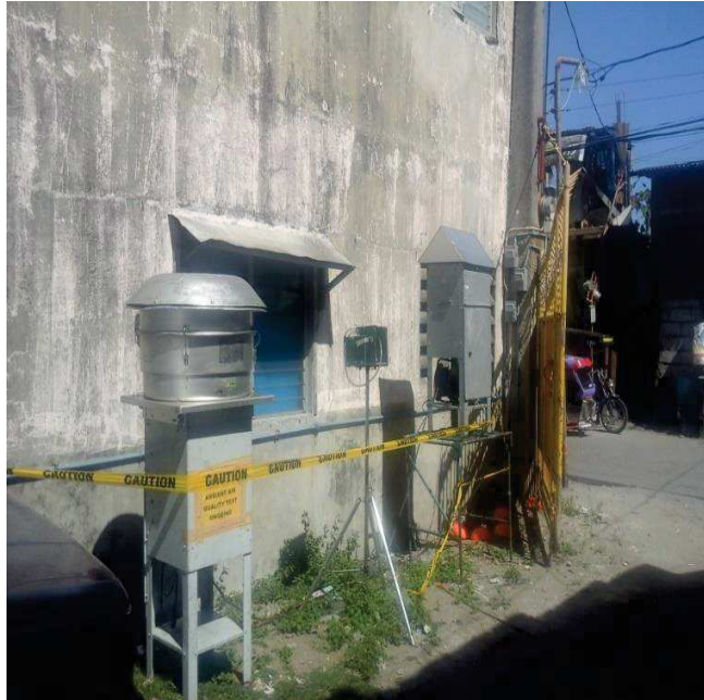
Figure 4.69 – Station A1, Sta. Rosa I, Noveleta
