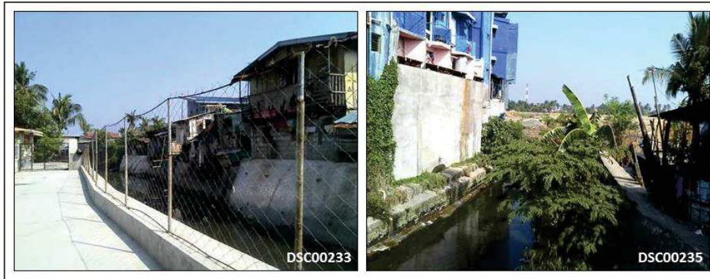
Figure 4.20: Narrowing of sections of waterways due to construction of residential houses along the Maalimango Drainage Improvement Project.
