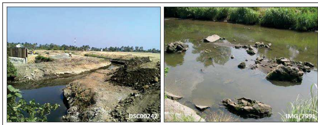
Figure 4.11: Construction excavation east of Maalimango River (left photo). Boulders of tuff breccia along Ylang-Ylang River Improvement Project (right photo).
