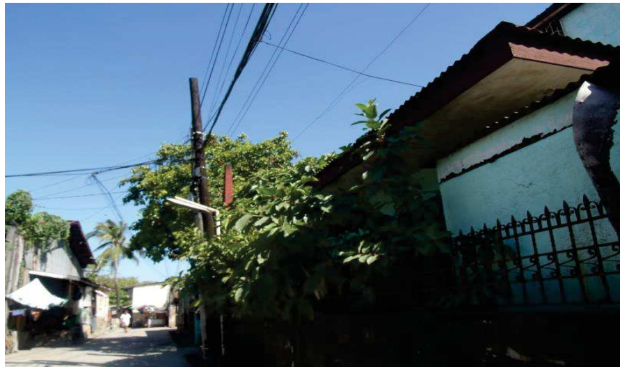
Figure 4.77: Sample photo of electrical connection (MERALCO) per household
