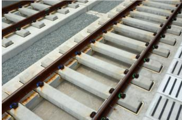
Figure 4.2.49 Ballast less Track structure (Elastic sleeper directly fastened track on concrete bed)
