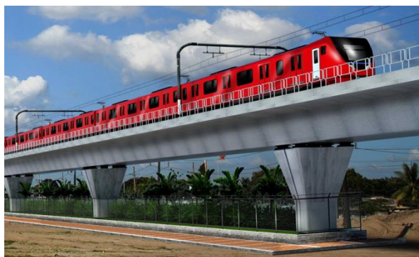
Figure 4.2.1 PC segmental box girder
