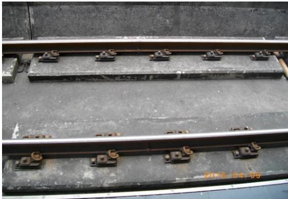
(i) Plinth Track
