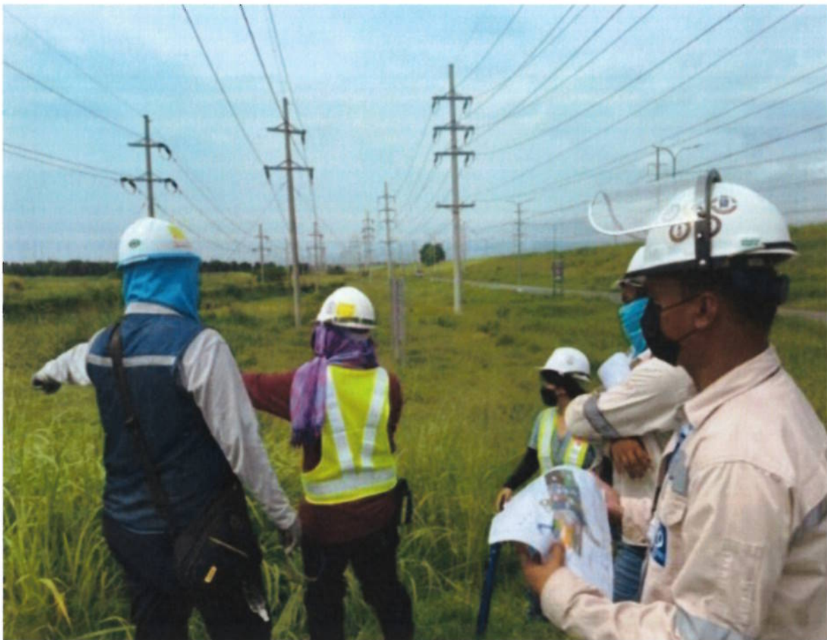
Location: : Drop Zone Area C Date: Sept. 6, 2021 Description/Comment: Site Inspection NW Drop Zone Permanent Access Road
