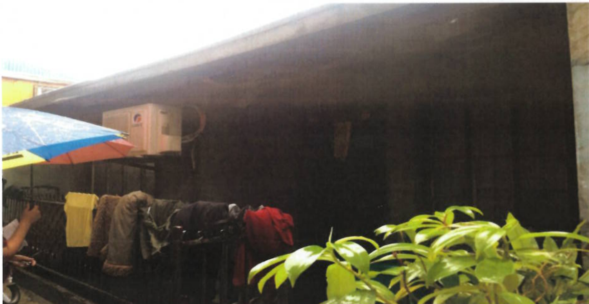
Location: Brgy. 348, Sta. Cruz, Manila, Metro Manila Date: July 28, 2021 Description/Comment: Inspection of NSRP-01-08-SN011, padlocked during sweeping because the SO was out of town
