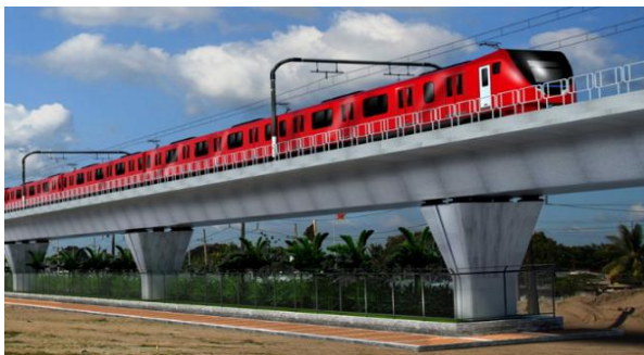
Figure 1.4.1 PC segmental box girder
