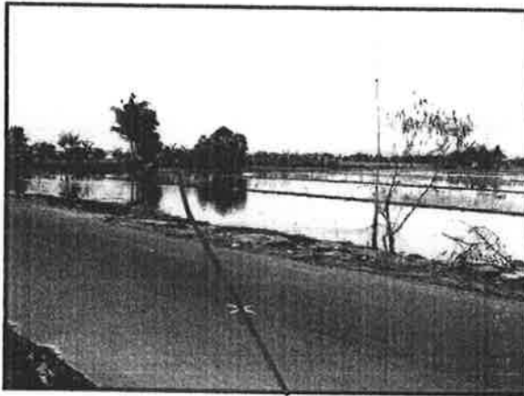
Plate No. 8 Taken at Sta. 5+564. Alignment crossing the Balagtas-San Jose Road in Brgy. Bulihan, Plaridel, (looking north).
