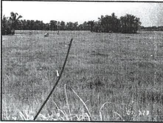
Plate No. 2 The alignment coming from Brgy. Borol 2nd, Balagtas crossing the open areas at Brgy. Tiaong.
