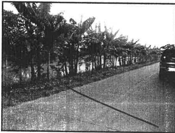
Plate No. 9 Taken at Sta. 7+653.15, looking south. Alignment crossing the Camachilihan-Liciada Road in Brgy. Camachilihan, Bustos.
