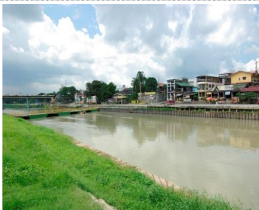
Marikina River Park, looking upstream. Commercial establishments are located on the left bank side.
