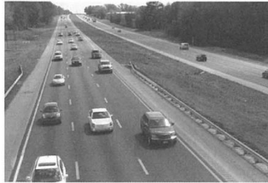
LOS E Operation at capacity
