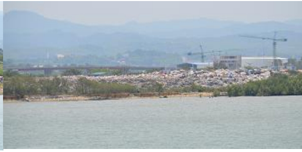
Opened Dumping Site
