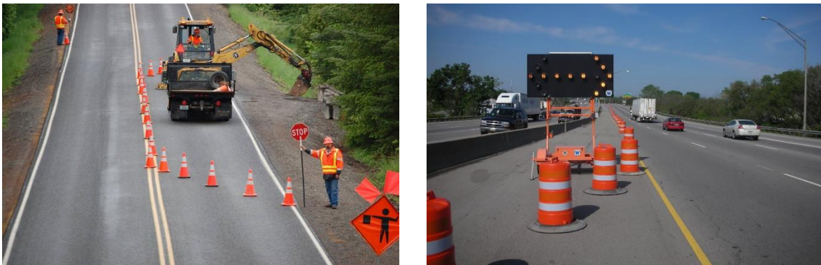
Figure 4.4.16 Images of Temporary Traffic Control
