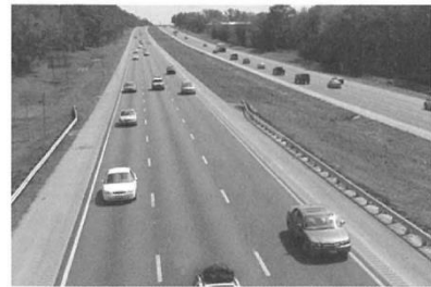
LOS C Flow with speeds near the free-flow speed of highway
