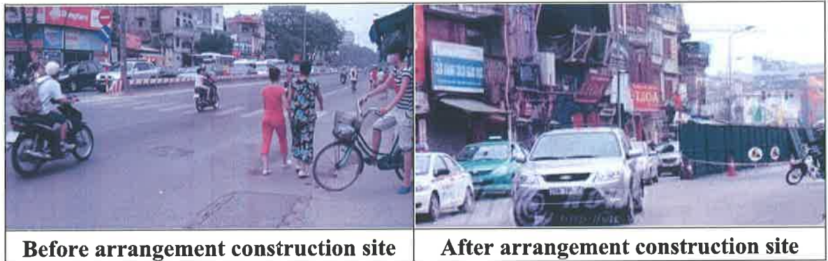
Figure 3.5 Illustrations the scope of traffic flow narrowed when construction site arrangement
