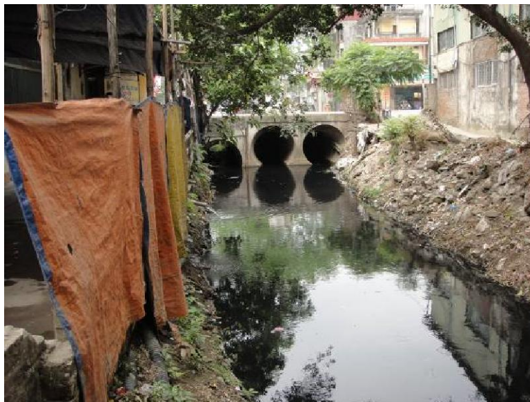
Figure 3.4. Drainage at Km2 +193
