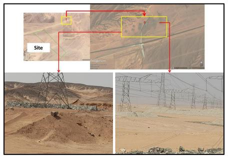
Figure 55: Stone and concrete fence at the base of the high voltages towers to protect them from surface run off.
