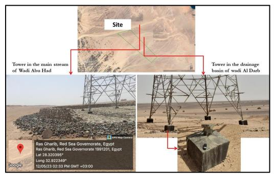
Figure 51: Mitigation measures to protect the tower of the power line running NNE- SSW to the east of the site.
