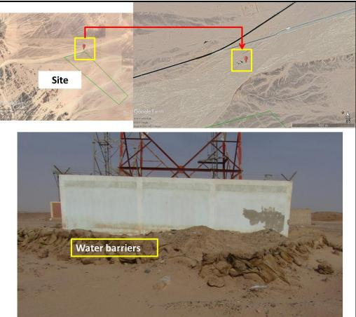
Figure 50: Containers (Shawwals) filled with sand and gravels stacked on top of each other, forming a wall about 1.5 meters high to protect the towers.
