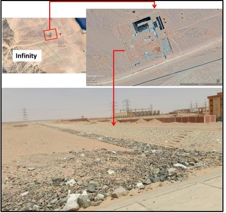
Figure 54: Stone and concrete fence protecting the power station.
