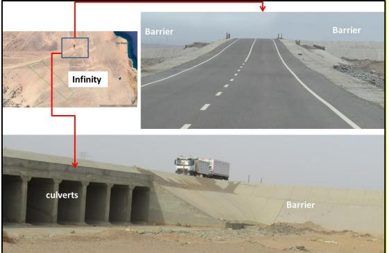
Figure 53: Field photographs show the water barrier at the km 8 and the associated culverts.
